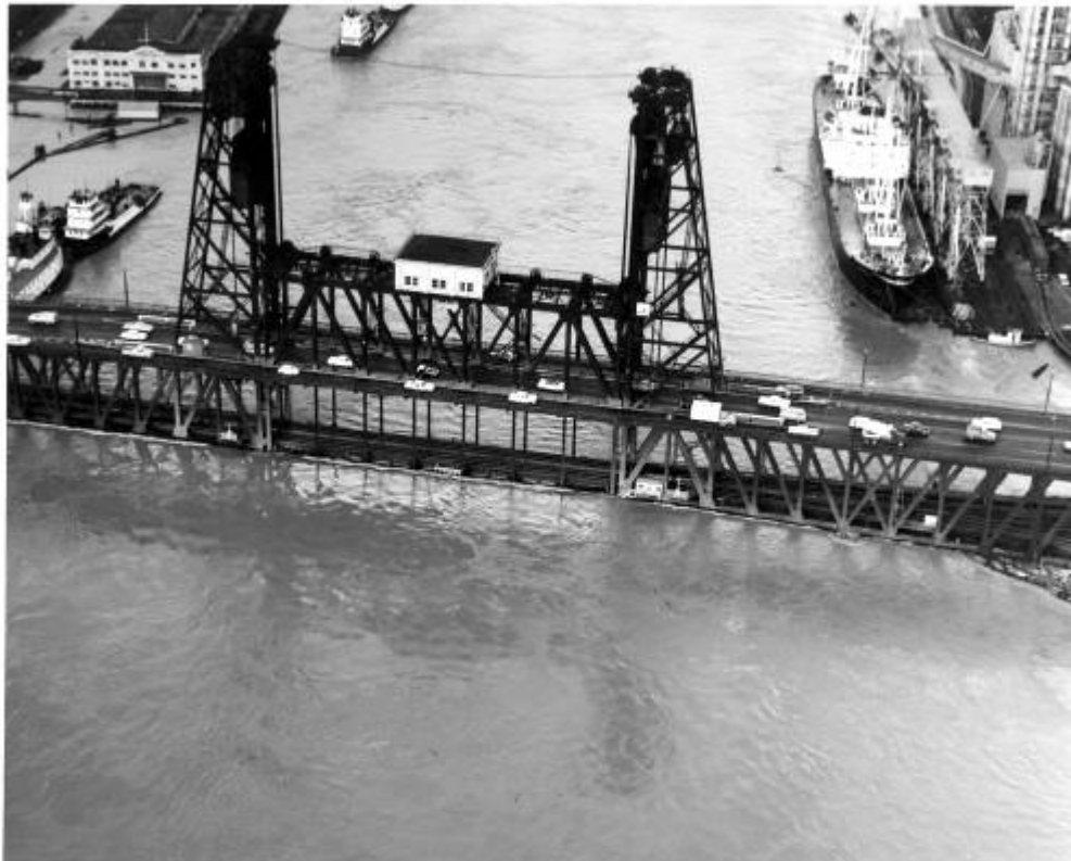
Photo Source: Oregon Department of Transportation
