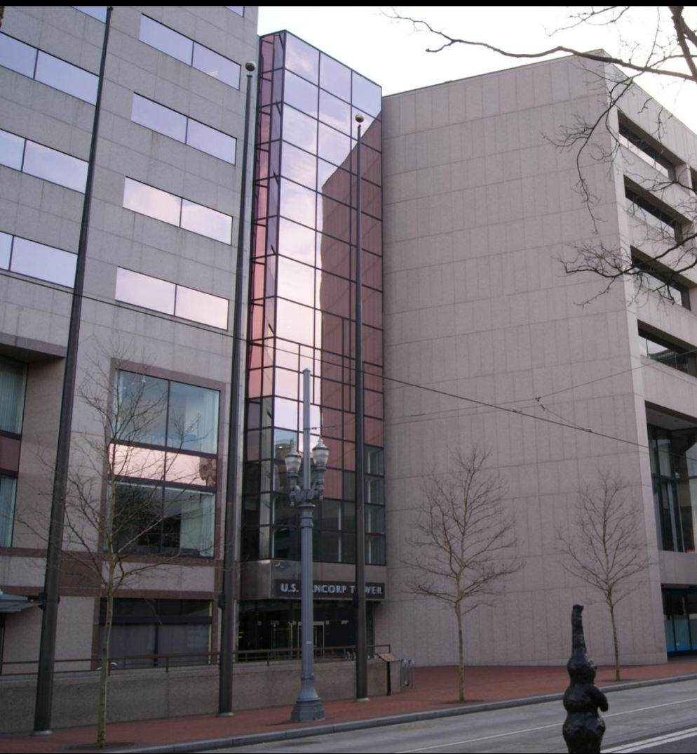
EXISTING WEST ENTRANCE
