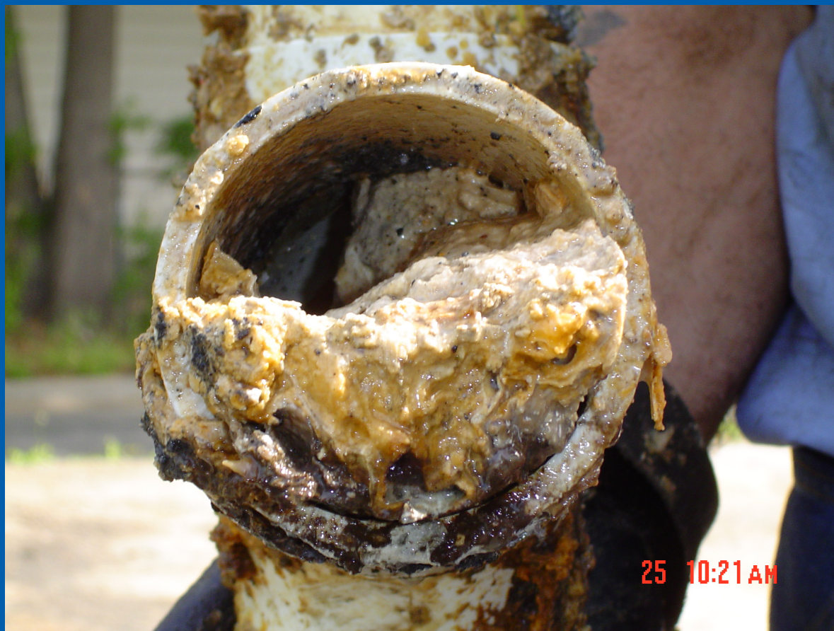
Line Replacement due to Grease Discharge
