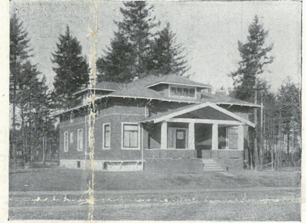
The home of Frank Schlegel in Rose City Park. It is located at the northwest corner of Coleman Avenue and the Alameda. Mr. Schlegel is a prominent Portland attorney with offices in the Worcester Block.
