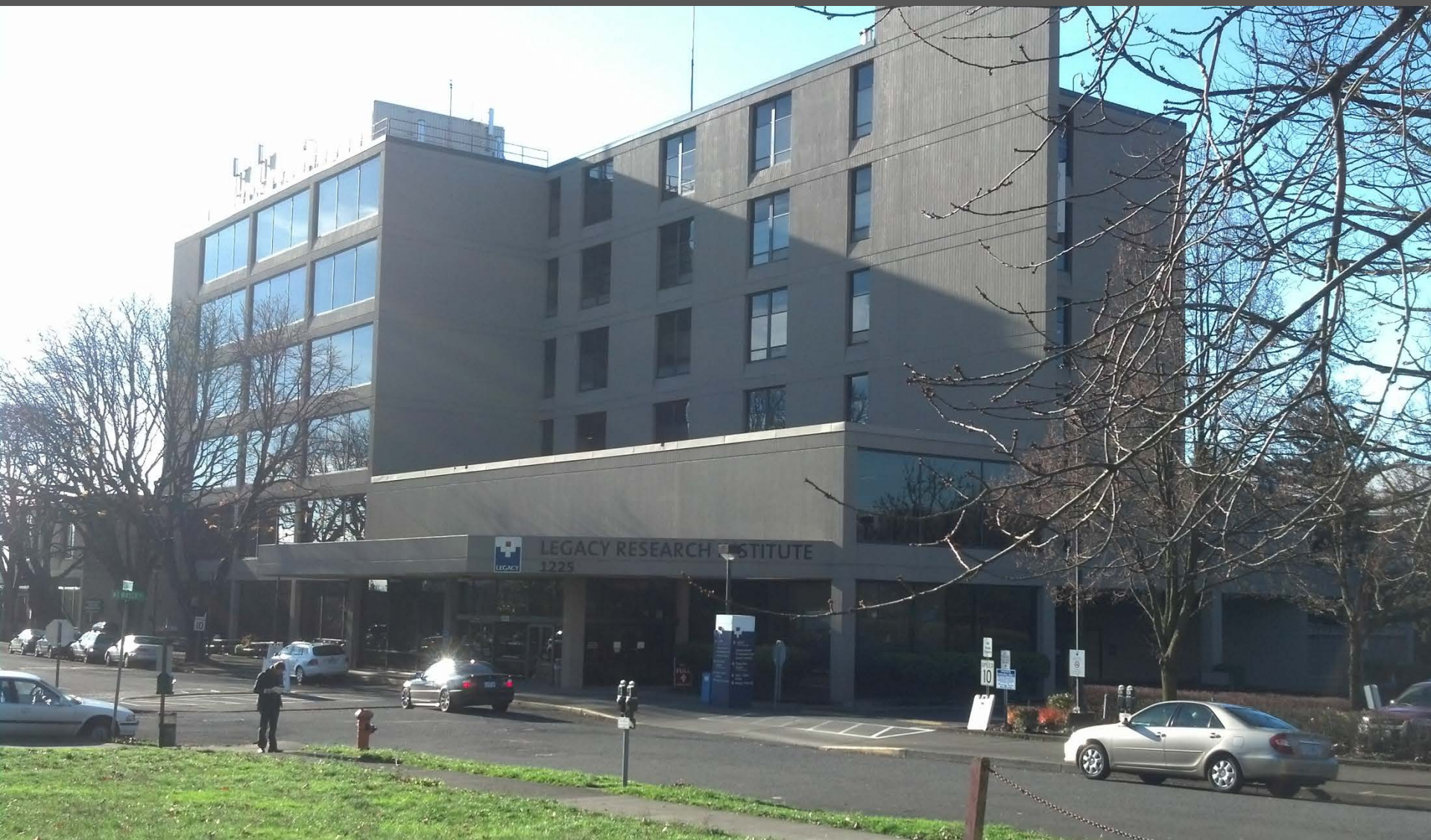
View looking southwest - Existing Lab Main Entry
