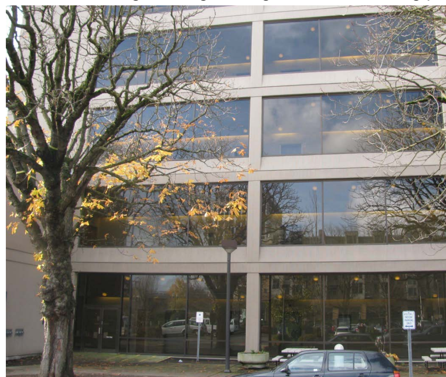
Existing east facade
