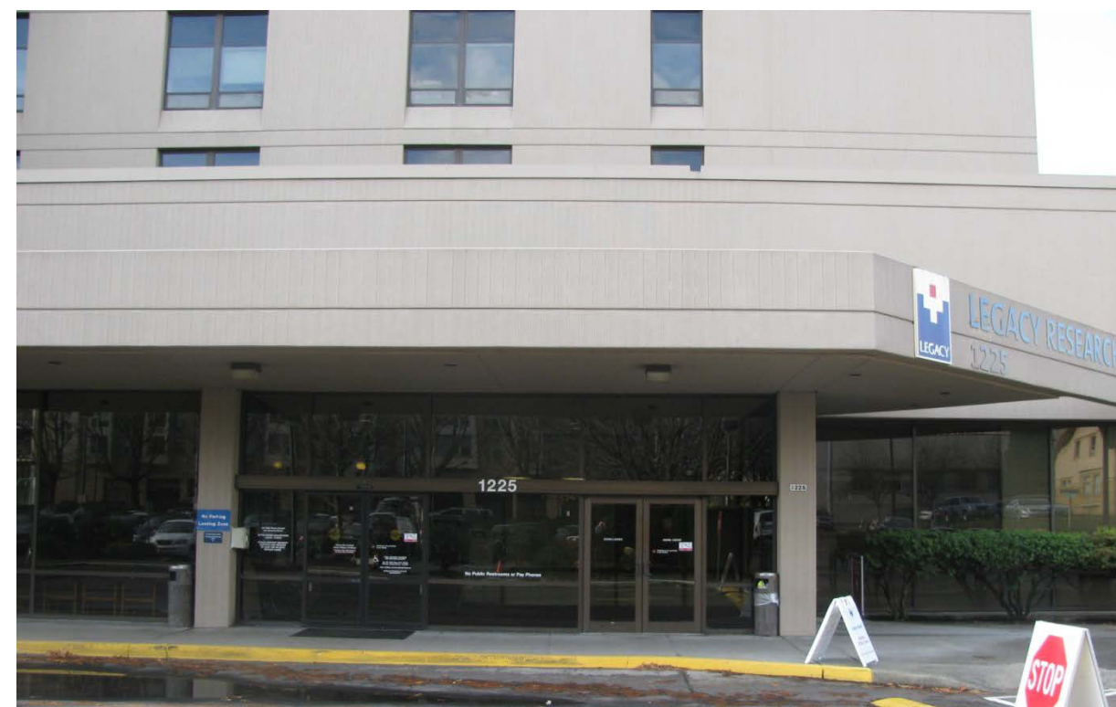
Main building entrance at NE 2nd and Wasco
