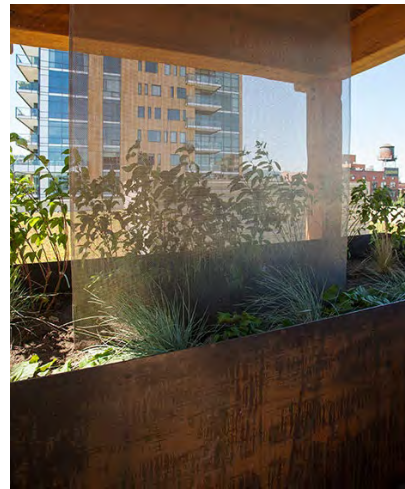
Rain Screen at Stormwater Planter
