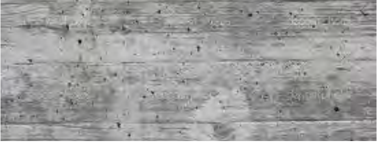
Board Formed Concrete
