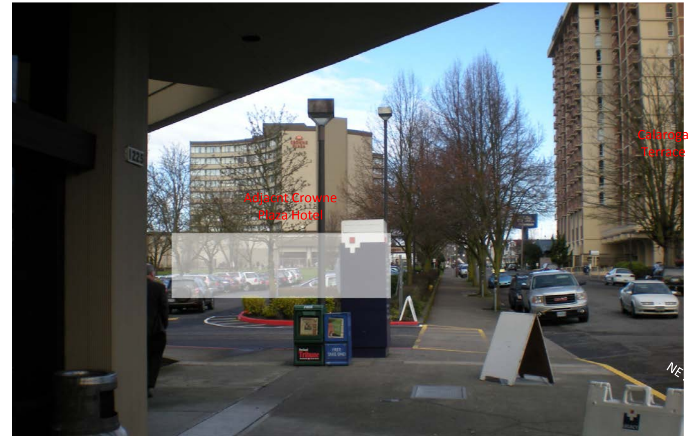
View looking north on NE 2nd from existing main building entrance
