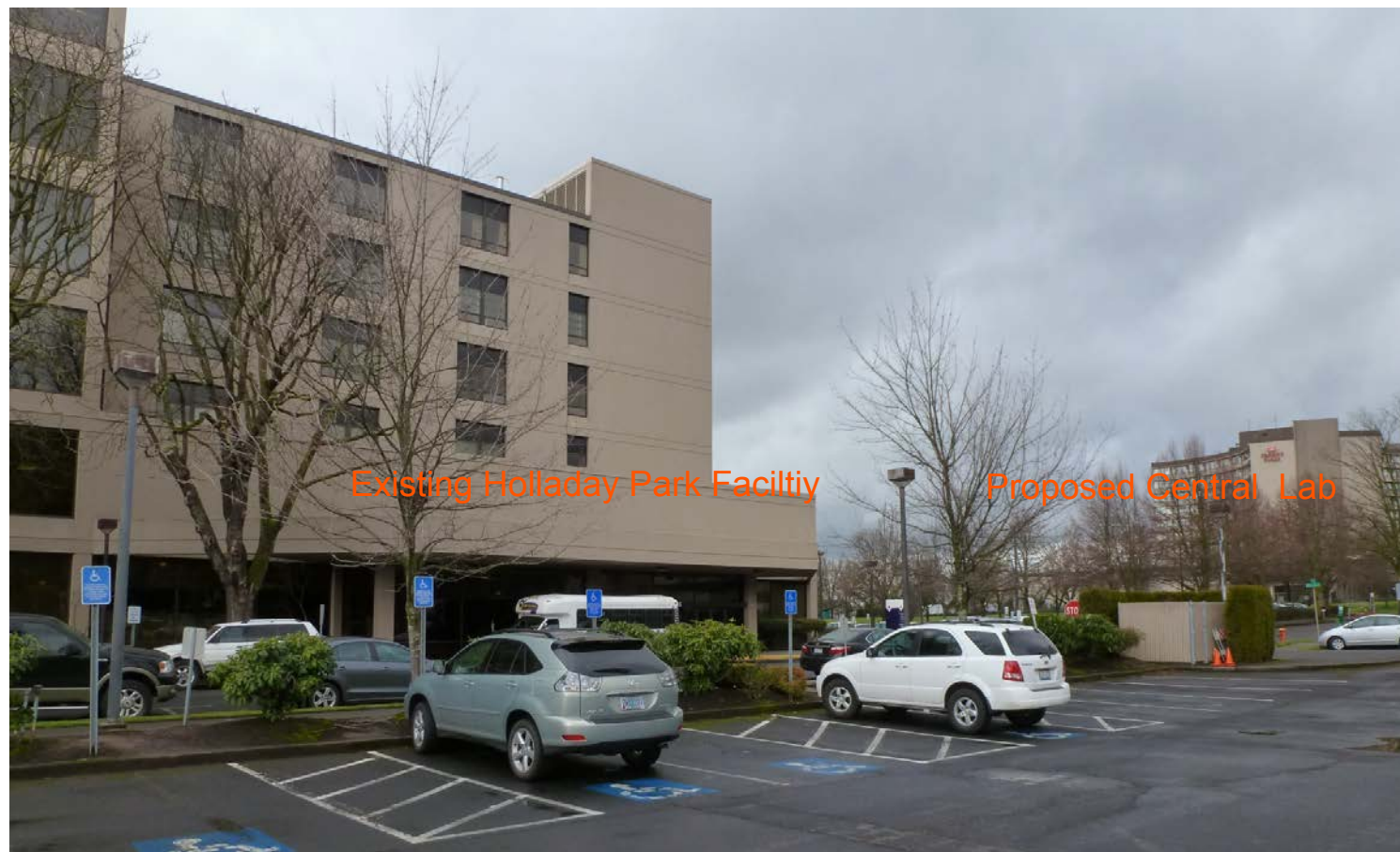
View of existing building looking west from existing parking lot
