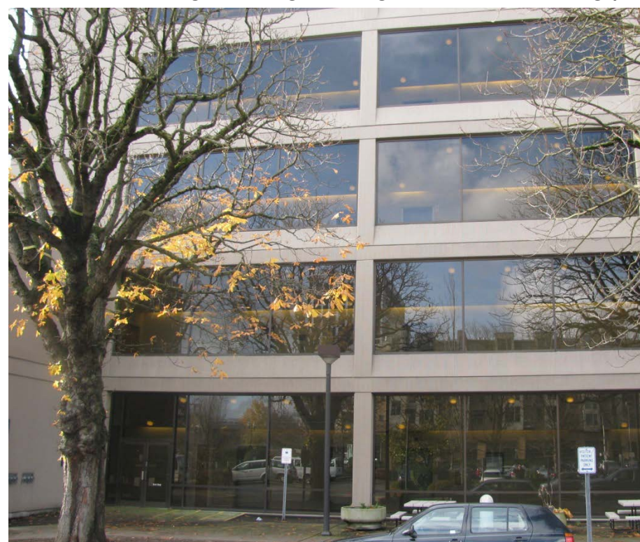
Existing east facade
