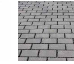
C. Permeable Pavers
