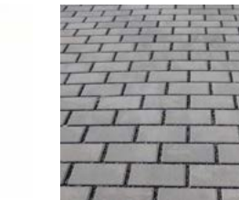
C. Permeable Pavers
