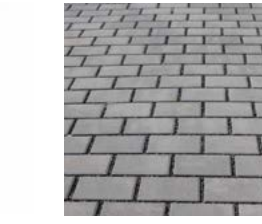
C. Permeable Pavers
