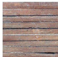
A. Board Form Concrete Stormwater Planter
