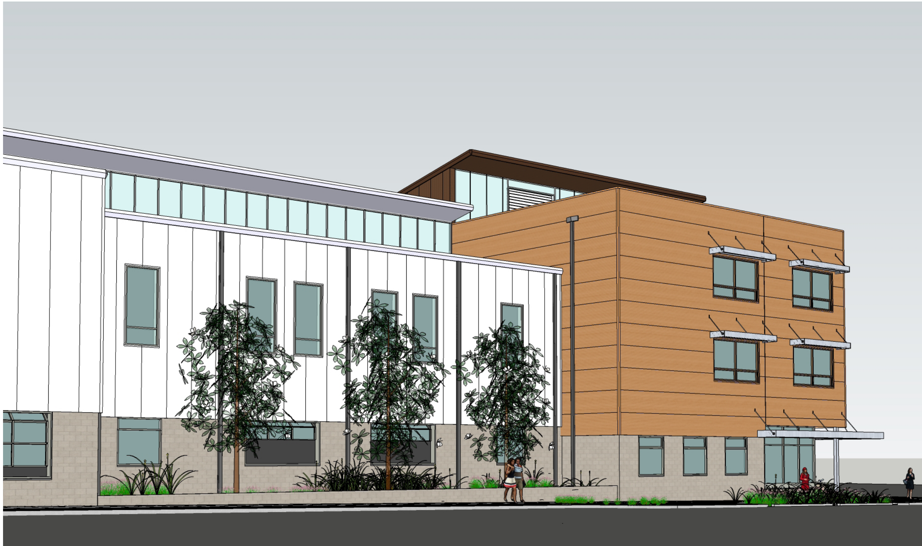
SOUTH CORNER VIEW
