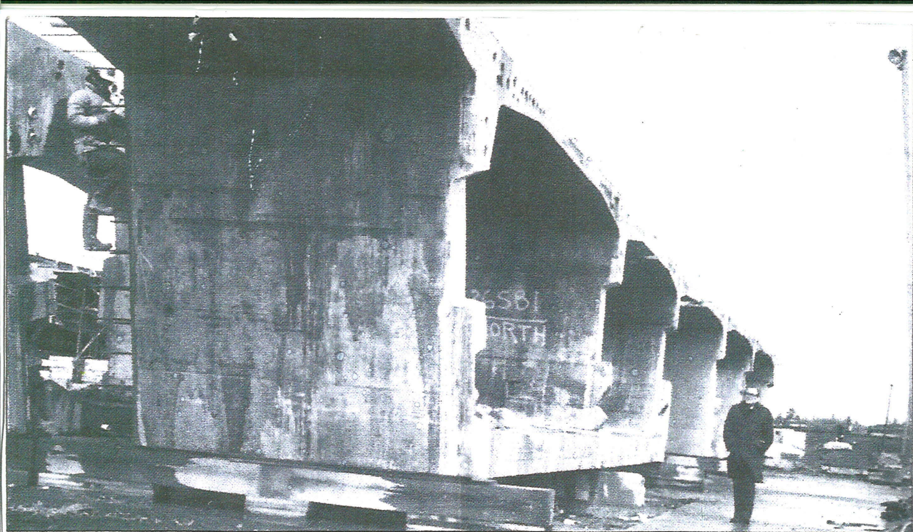
Several of 592 precast-concrete segments are shown here in the yard. The precast segments were produced in 12-foot, 15-foot, and 17-foot depths at a location four miles downstream. The segments were temporarily held in place by high-strength threaded rods. Once all segments were in place, tendons were installed in the ducts, visible near the top, and post-tensioned.
