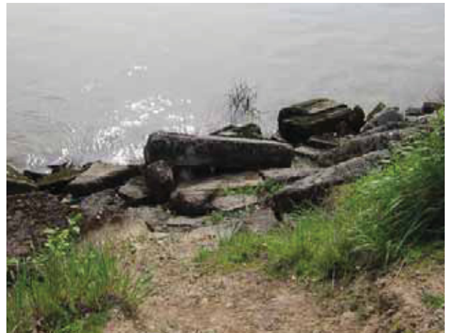
Existing demolition debris and large unstable concrete pieces
