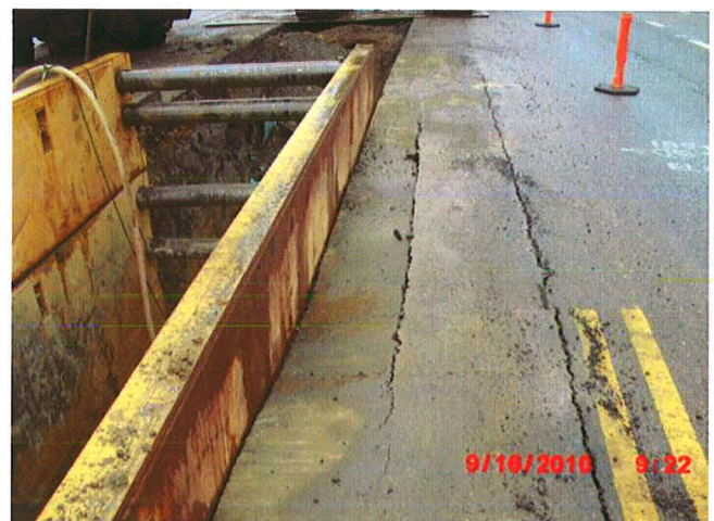
PAVEMENT CRACKING OUTSIDE TRENCH
