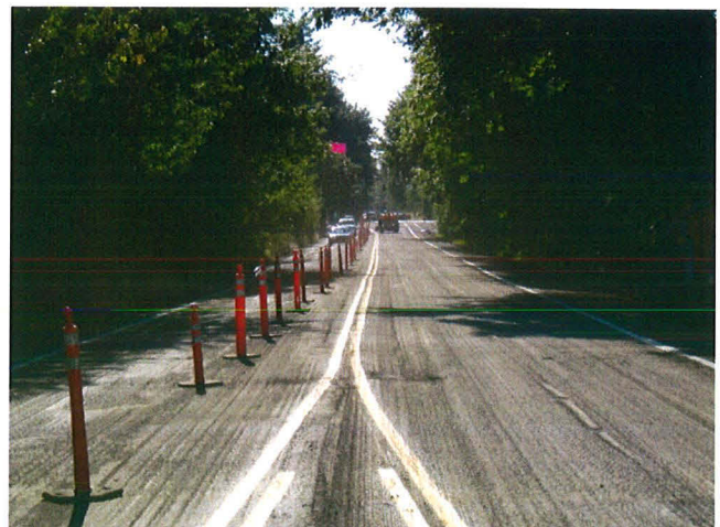
GRINDING ROAD FOR GRIND & PAVE
