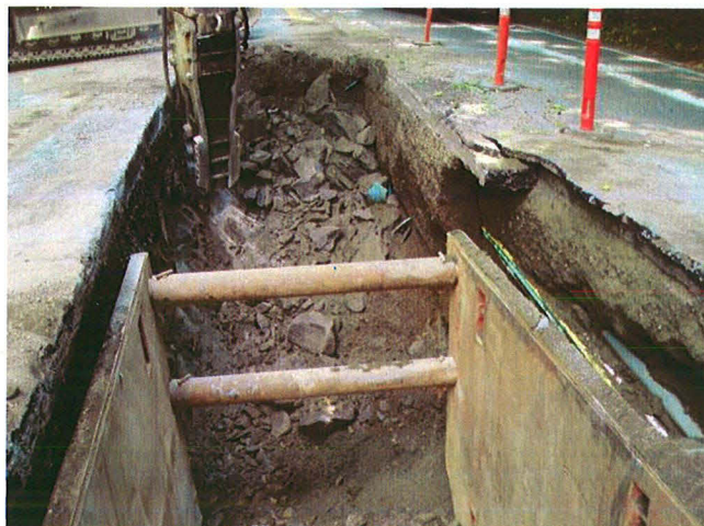
TRENCH ROCK EXCAVATION
