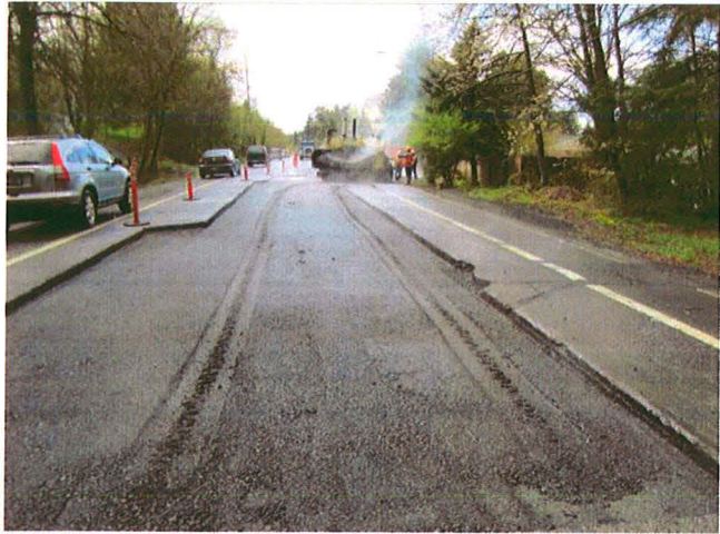
8" AC PAVING OVER FORCE MAINS
