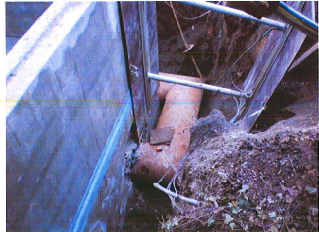
TEMPORARY OUTLET PIPE AT DISCHARGE STRUCTURE
