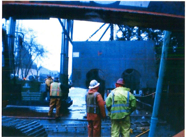
SETTING DISCHARGE STRUCTURE @ 31 ST & MULTNOMAH
