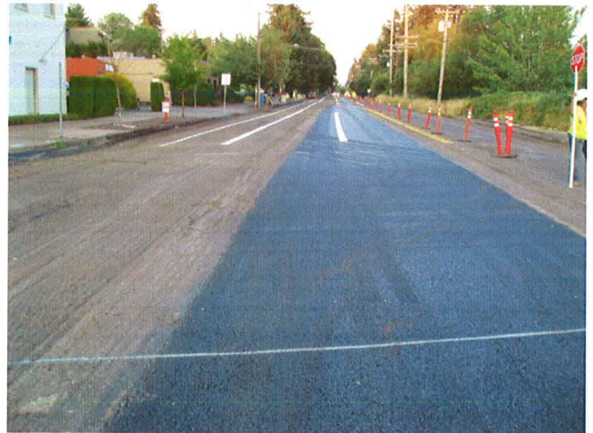
GRIND & PAVE TRENCH PATCH AT SW 40 TH
