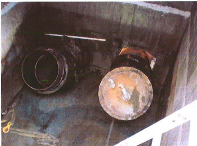
"B" LINE WITH CAP IN DISCHARGE STRUCTURE
