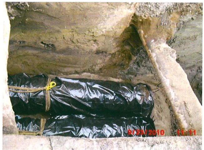
WRAPPED FORCE MAIN PIPES
