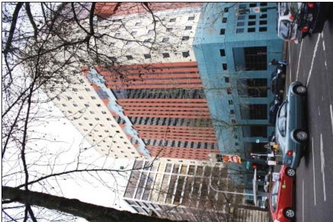
Photo 6 of 11: OR_MultnomahCounty_PortlandPublicService_0006.tif South facade (right) and east facade (left), looking northwest.
