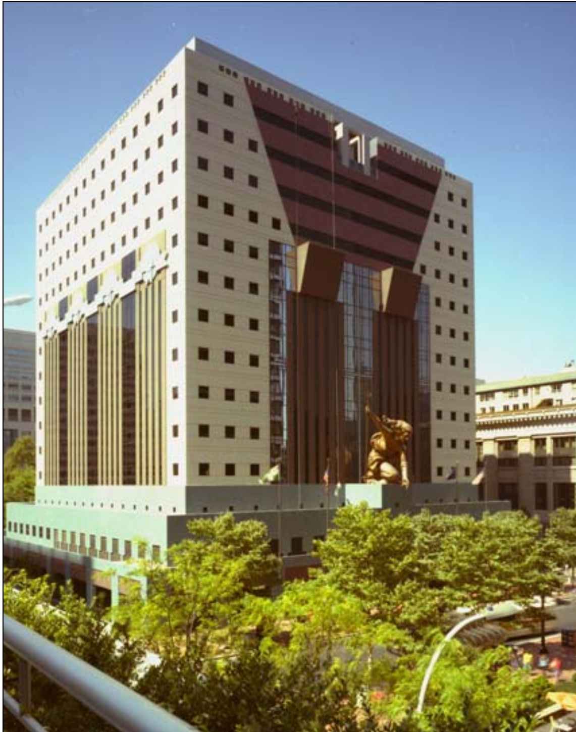
Figure 8: West side of the Portland Building, photo dated 8/19/1986 From the City of Portland archives
