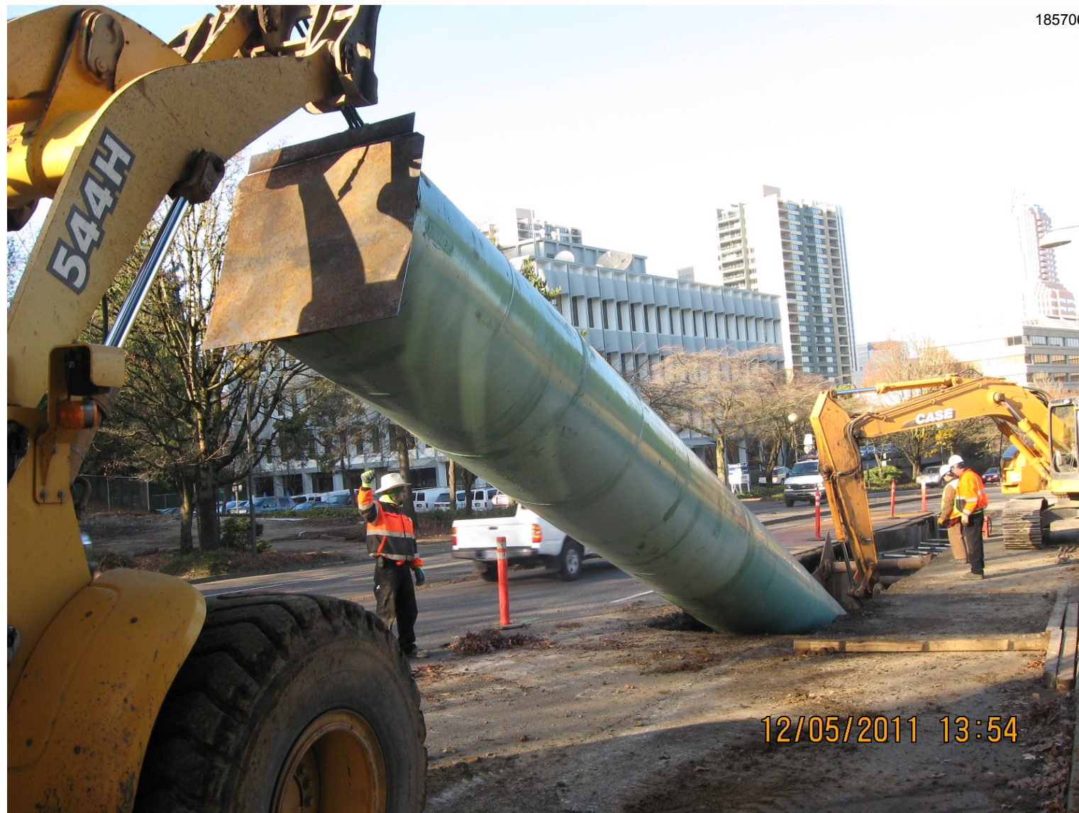
Installation of 48" diameter steel casing under the future SW Lincoln Street and the new light rail line on SW Naito Parkway.
