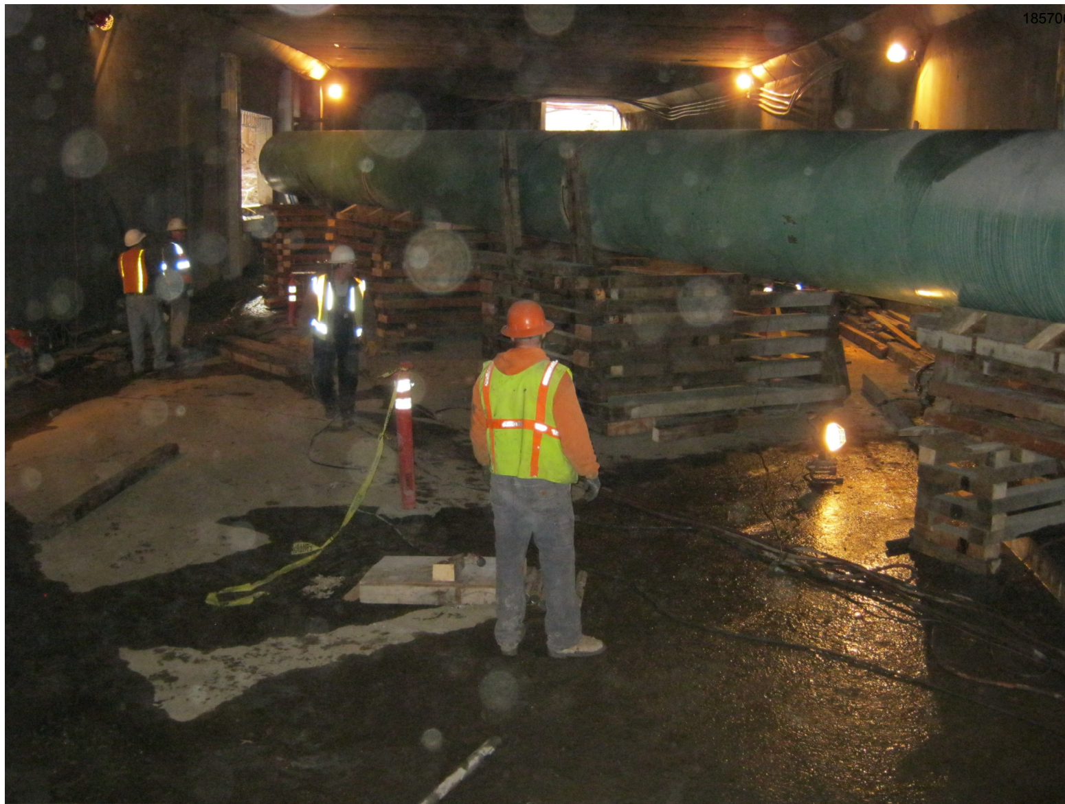
Pulling the 48" steel casing through the Grant Street tunnel.
