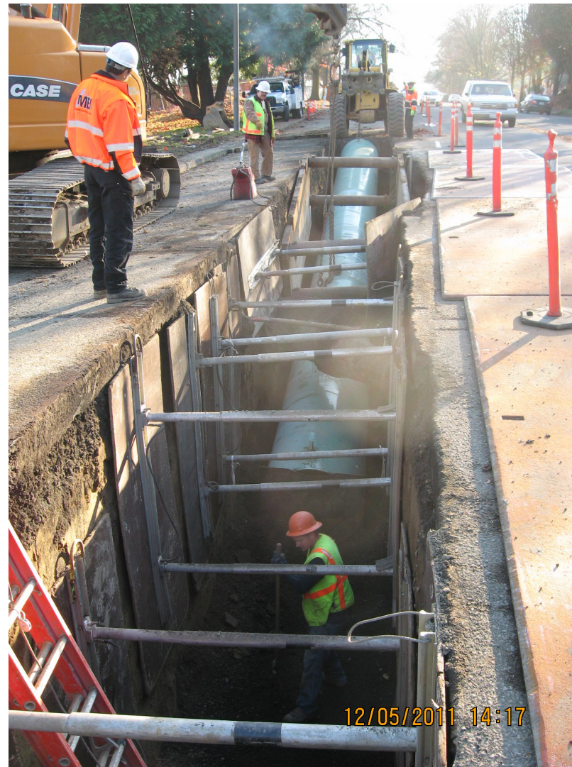
Installation of 48" diameter steel casing under the future SW Lincoln Street and the new light rail line on SW Naito Parkway.
