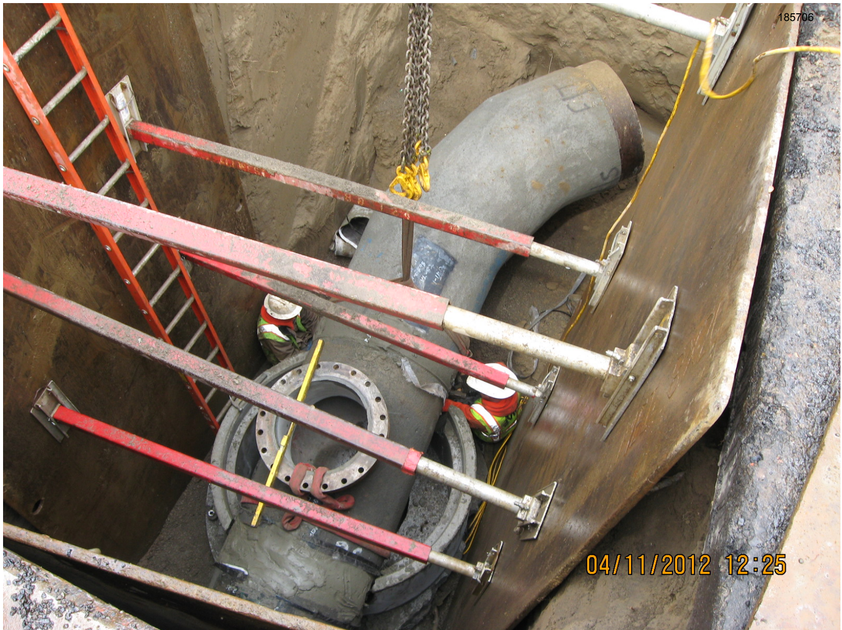
Setting manway at SW 1st and Porter (to tie into Phase 1). Depth = 14 feet
