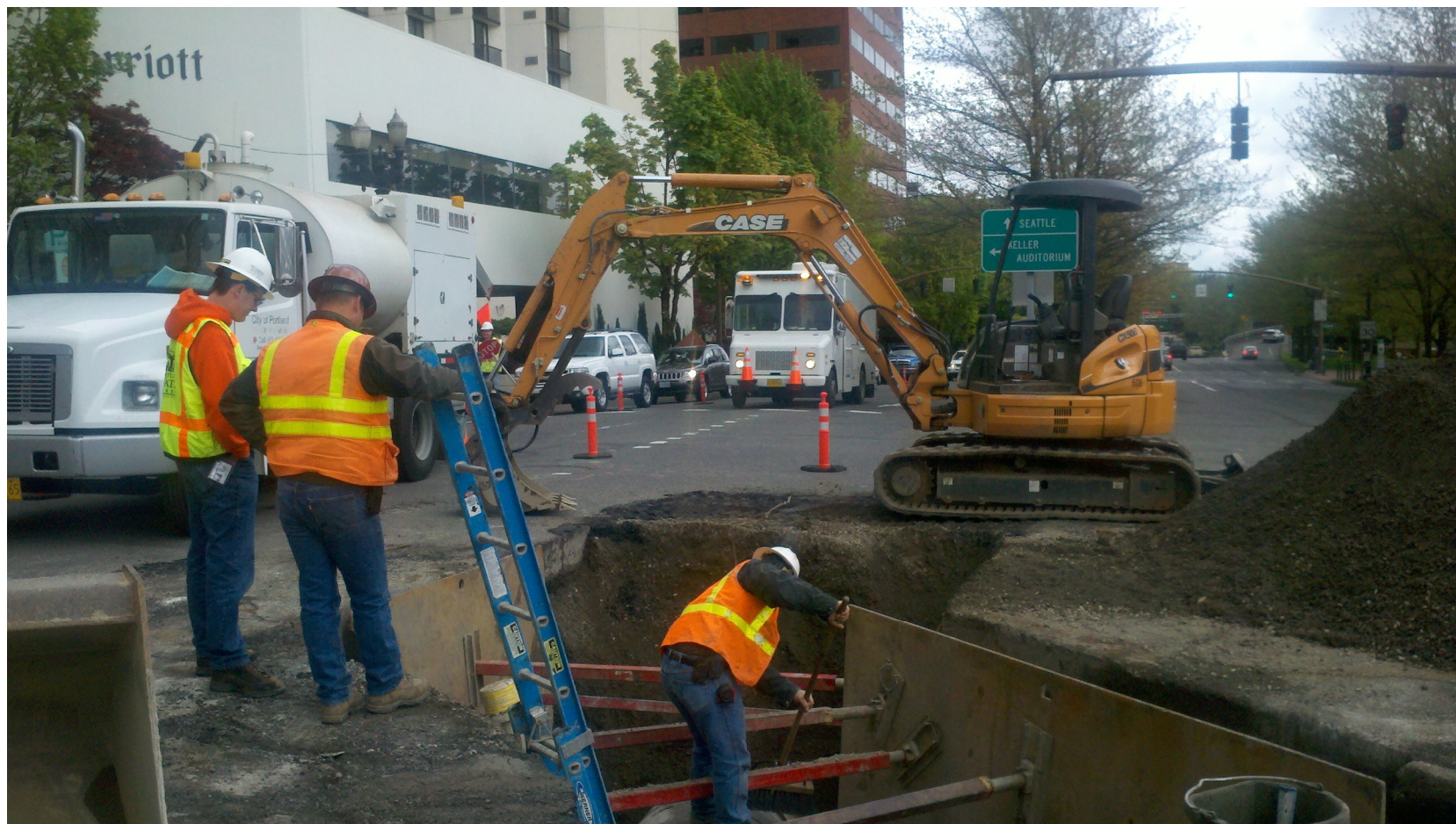
SW Clay and Naito tie-in. BOM on site helping clear out catch basin to discharge into for testing
