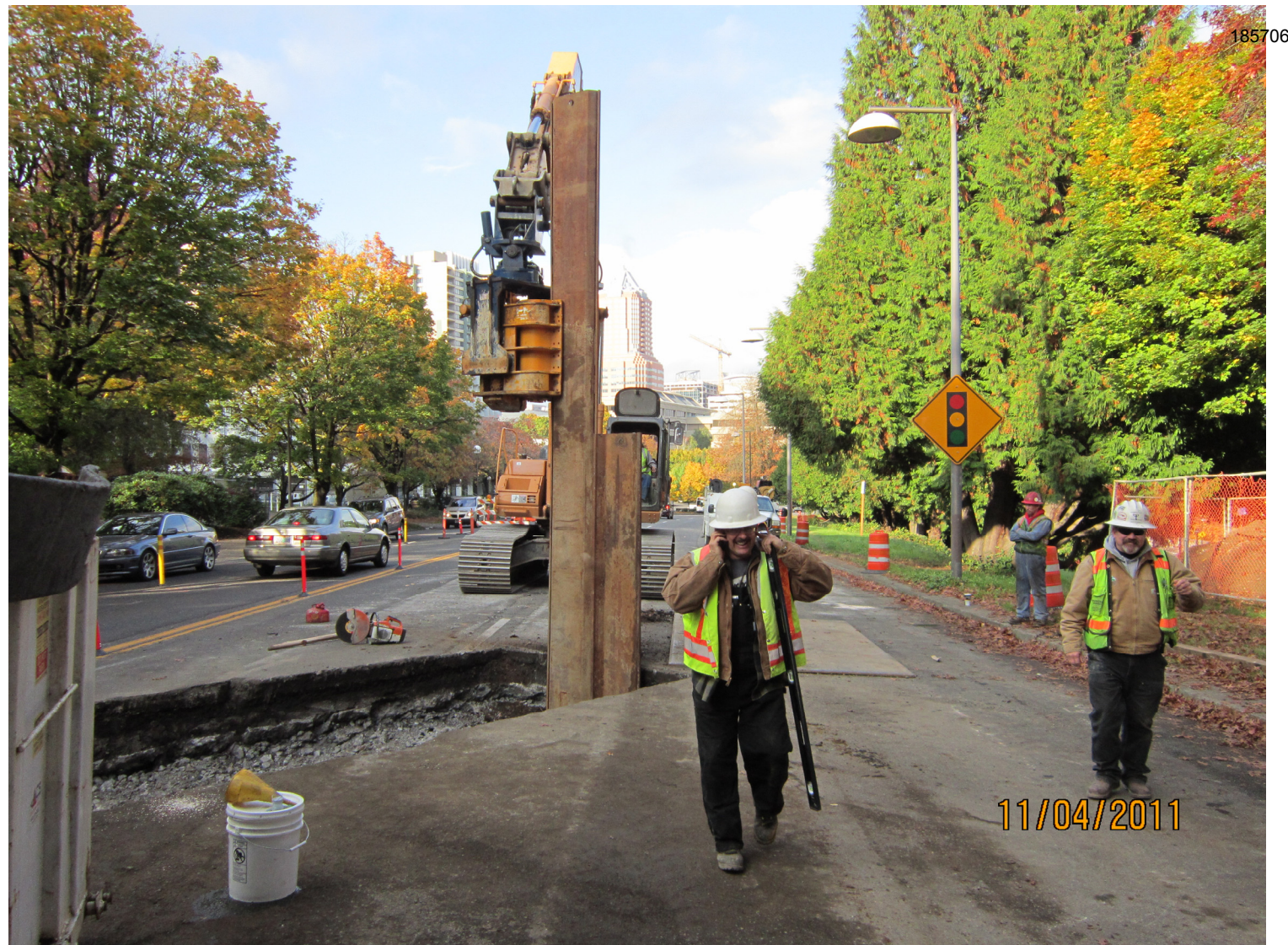
Contractor installing sheet piles in SW Naito Parkway on the exterior tunnel walls. The will provide support when the 40" and 24" casings are pulled through the tunnel walls.
