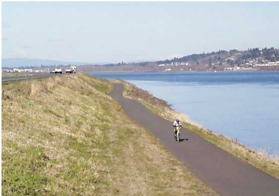
Figure 5.2 NE Marine Drive Levee
