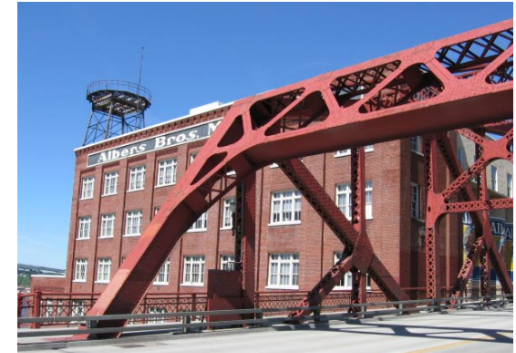
exterior of the Albers Mill building today
