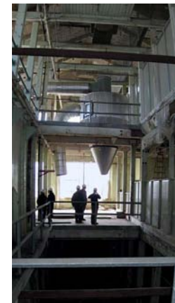
Feed Mill interior
