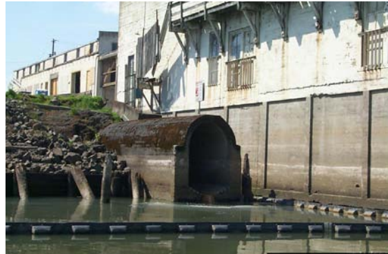
Tanner Creek outfall (photo: Flowing Solutions)
