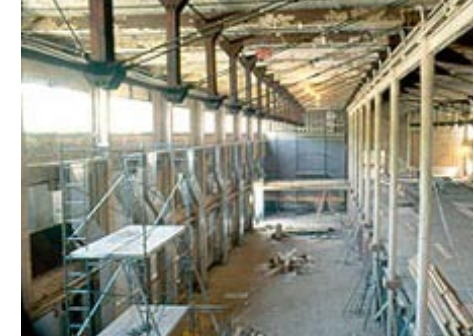
interior before renovation
