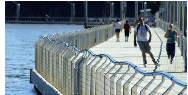
floating concrete walkway (Brisbane, Australia)
