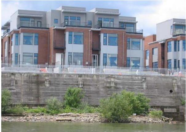
Willamette River seawall with adjacent development (photo: Flowing Solutions)
