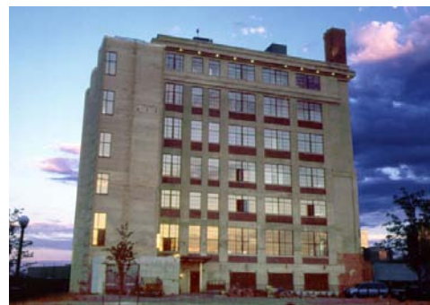
Flour Mill Lofts exterior
