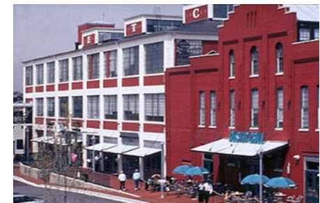
exterior of building after renovation
