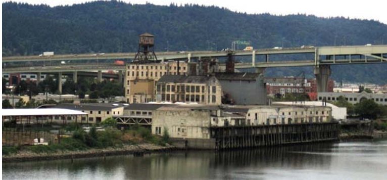
Centennial Mills as seen from the Broadway Bridge
