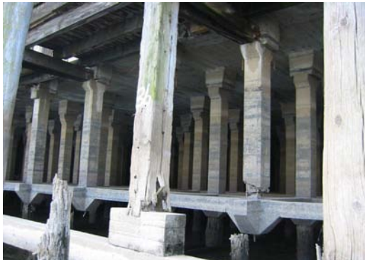
existing pilings (photo: Flowing Solutions)
