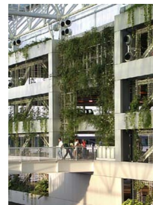
parking garage, Portland International Airport (Portland, OR)
