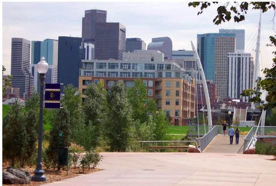
pedestrian bridge (Denver, CO)
