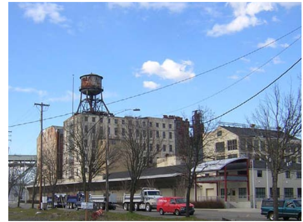
Centennial Mills as seen from 9th Avenue
