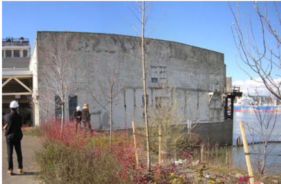
view of riverbank, southern edge of Warehouse C
