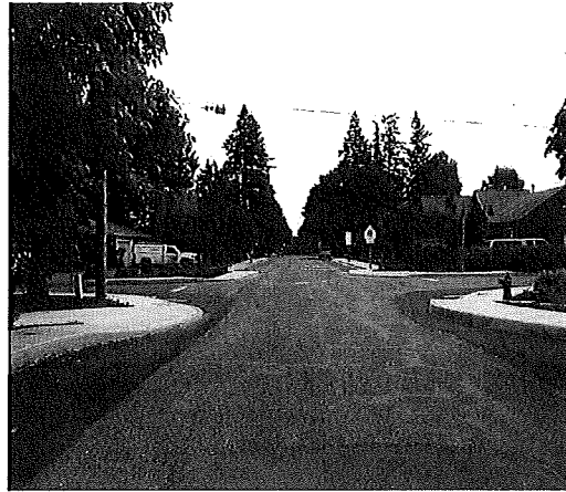
New sidewalks on the north and south side of Main Street between Third and 214 th Streets, west of the Elementary School, included installation of traffic calming corner bump-outs.
