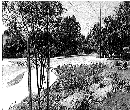
Project included rain gardens—a low impact development technique for stormwater management.
