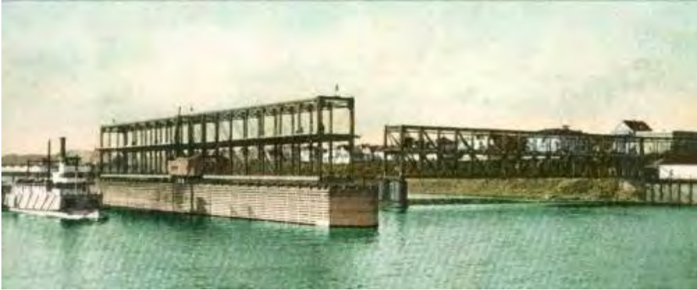
First Steel Bridge, 1888
