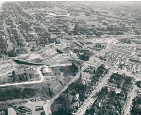
I-5 construction near Broadway/Weidler, 1962. Paramount Apartments and Leftbank Building at center
