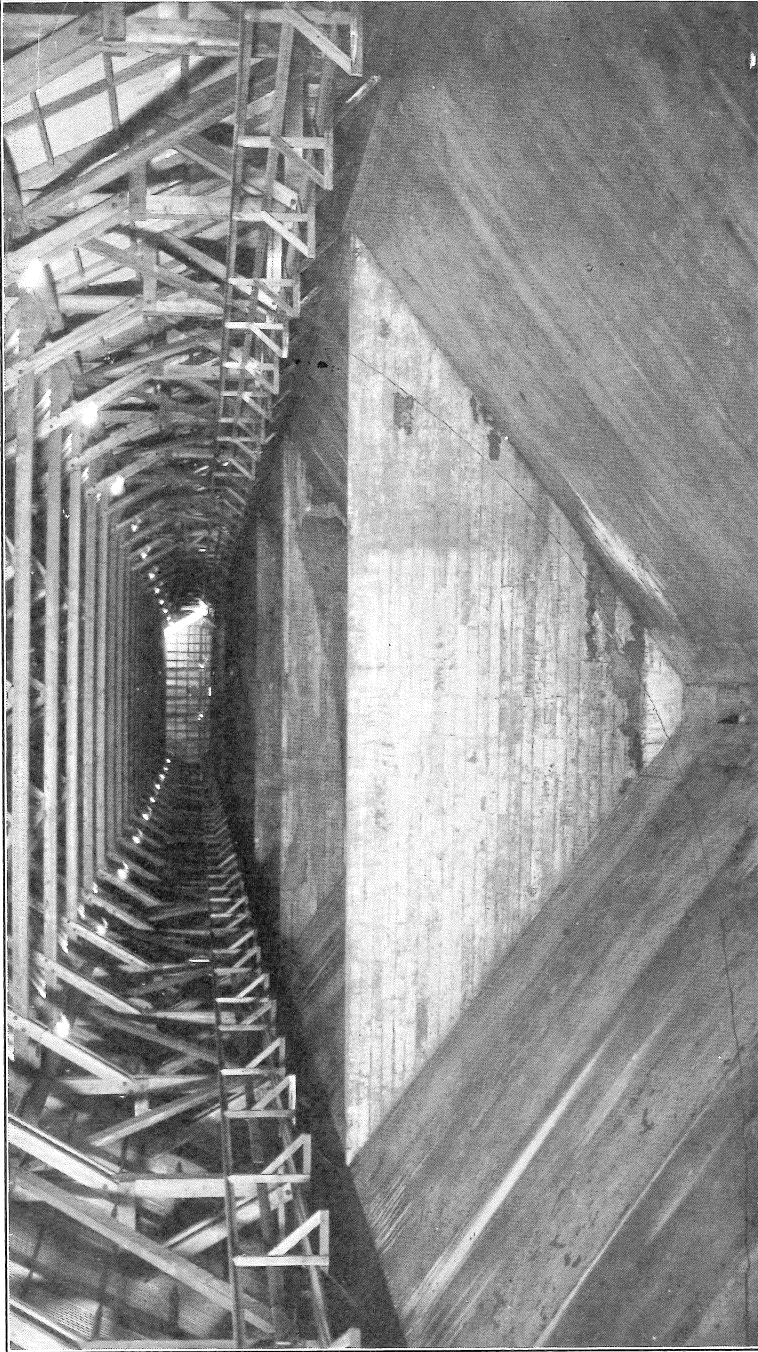
INTERIOR OF STORAGE BUNKERS OF BULK STORAGE PLANT AT PORTLAND MUNICIPAL TERMINAL NO. 4 The Bunkers Are of Reinforced Concrete Construction
