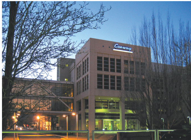
One of Con-way's two office buildings in Northwest Portland.
