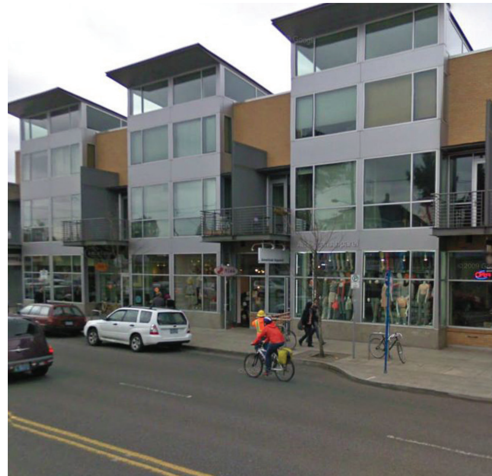
This building in southeast Portland takes up a full city block face, but has multiple narrow retail storefronts to help create diversity and interest along the street.
