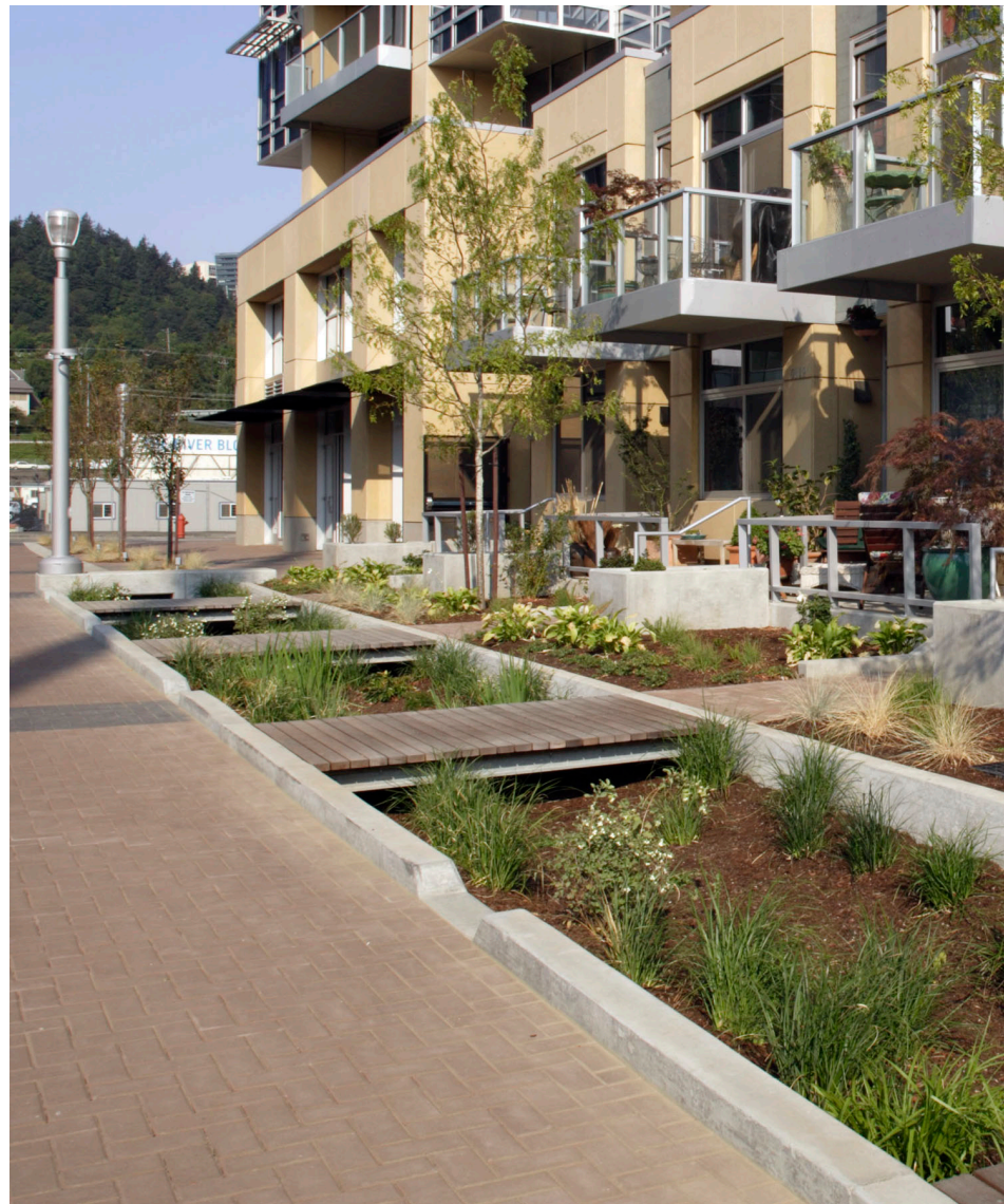
5. This image is of a landscaped pedestrian accessways in the South Waterfront. The swale and movement paths on either side give an indication of a stormwater design that could be developed within pedestrian accessways.
