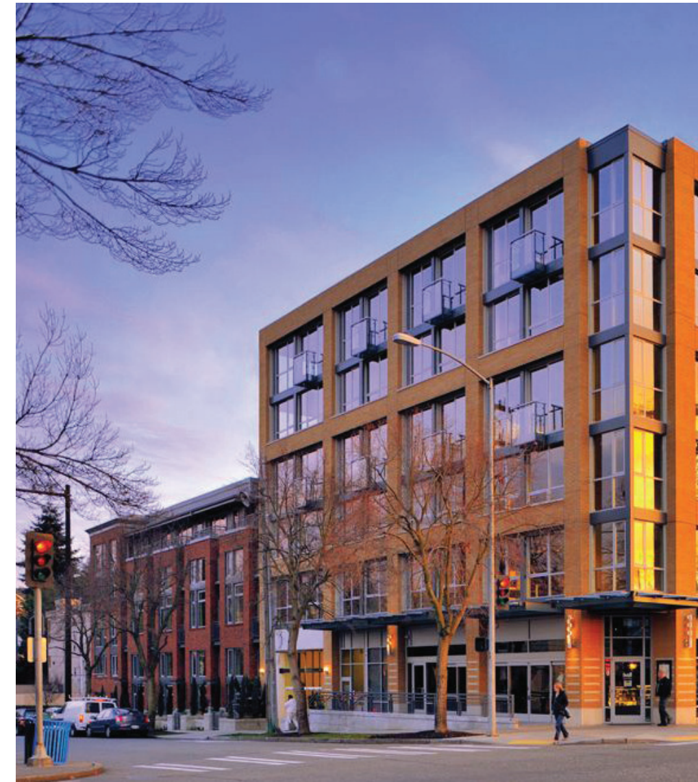
This is one large development that has been successfully articulated as different building volumes. The buildings are articulated using different heights, as well as a change in materials.
