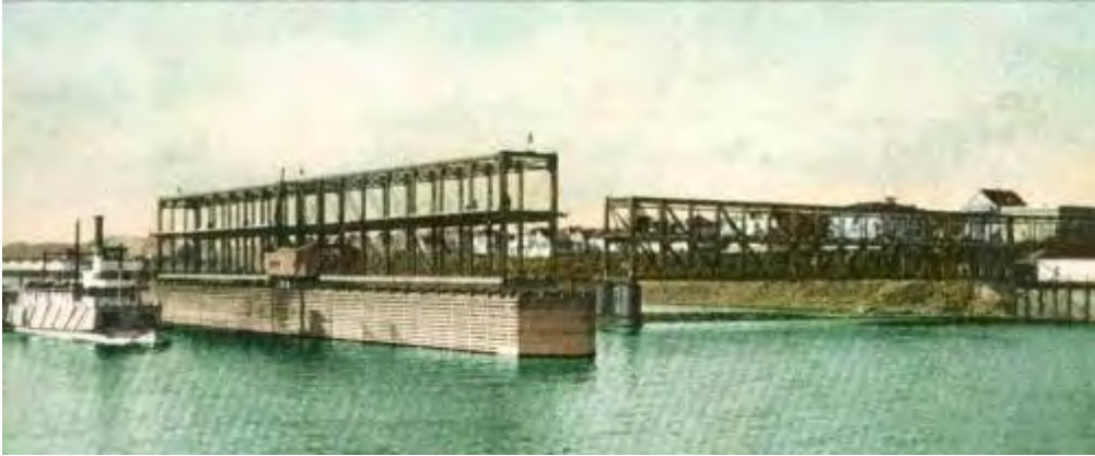
First Steel Bridge, 1888
