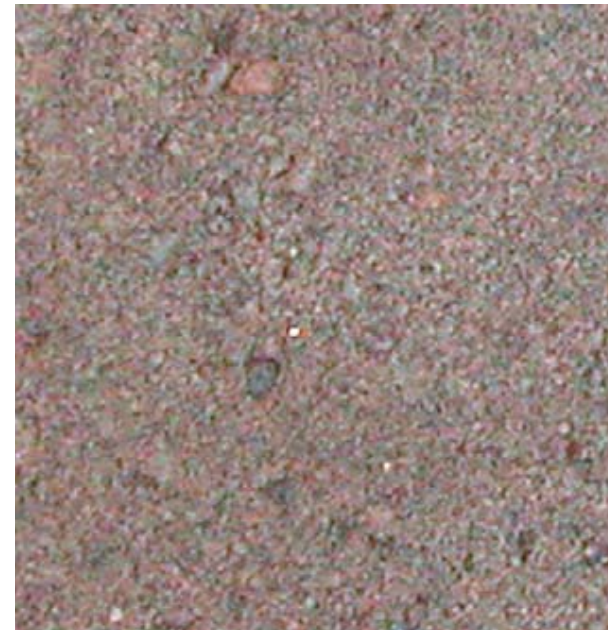
Light Colored Concrete
