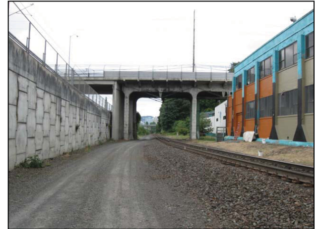
Building near railroad tracks east of NE 28th Avenue
