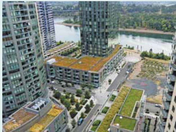
Ecoroofs help manage stormwater and bring nature into the South Waterfront area.
