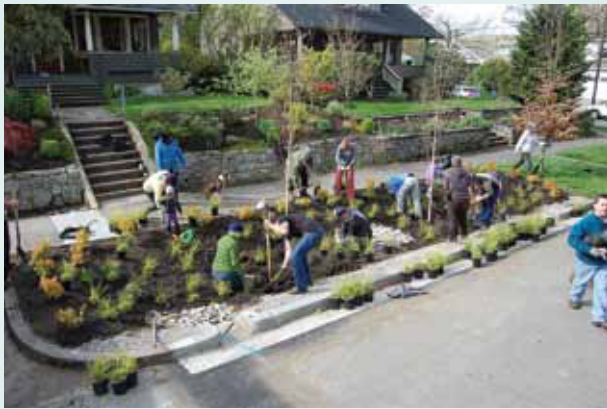
Vegetated green street facilities in the Tabor to the River area will help reduce pollution and basement flooding.
