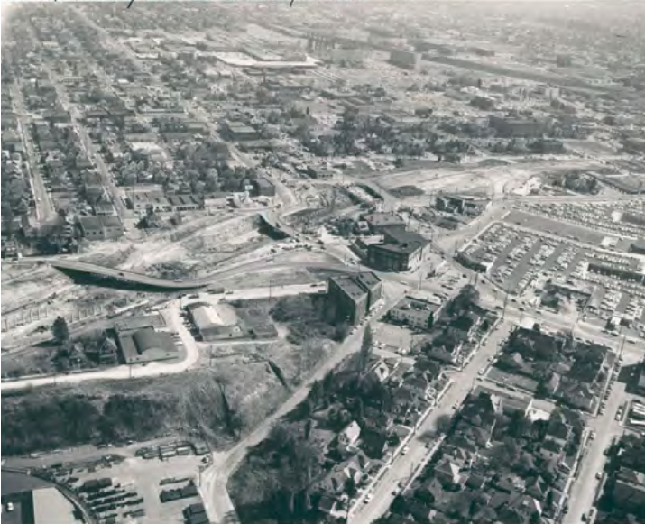
I-5 Construction near Broadway-Weidler, 1962, Paramount Apts. & Leftbank bldg. at center
