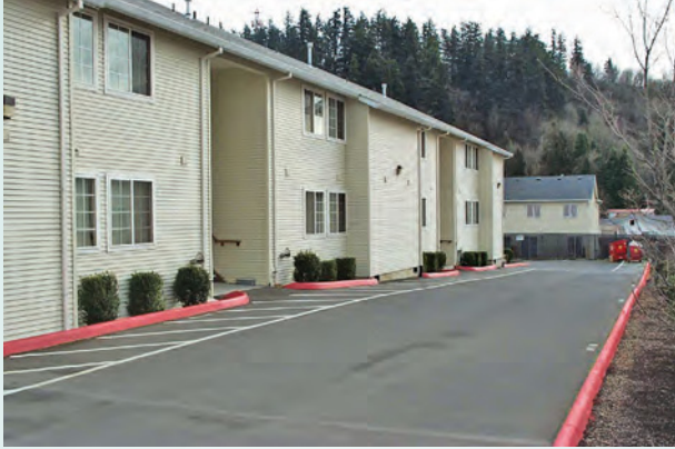
Driveway paved using conventional methods and materials.
