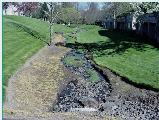
A no-build drainage reserve area runs through a multifamily residential development.
