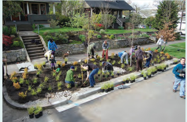
Vegetated green street facilities in the Tabor to the River area will help reduce pollution and basement flooding.
