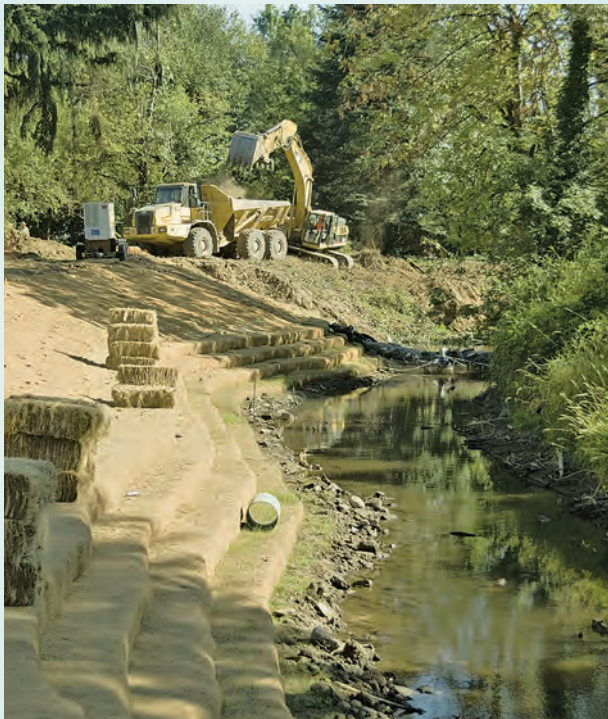
Acquisition of frequently flooded properties reduces hazard risk and allows restoration of East Lents section of Johnson Creek.
