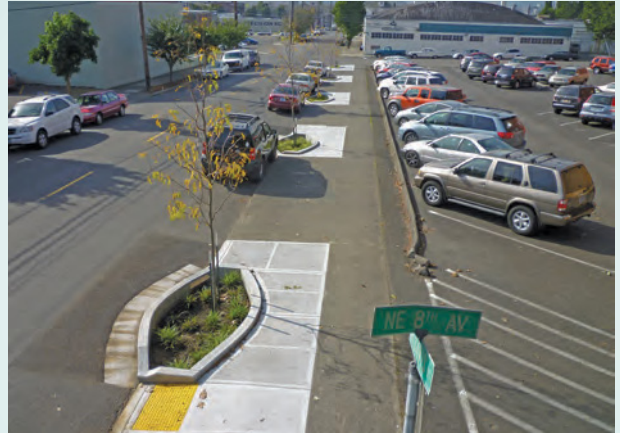
Innovative green street designs bring nature and stormwater management into the Central Eastside Industrial District.
