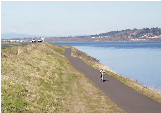
Figure 5.2 NE Marine Drive Levee
