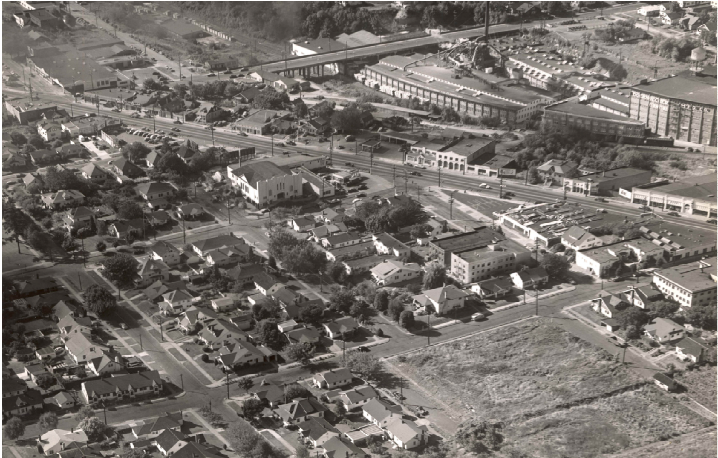
NE Sandy to 28 th St. Viaduct 1947
