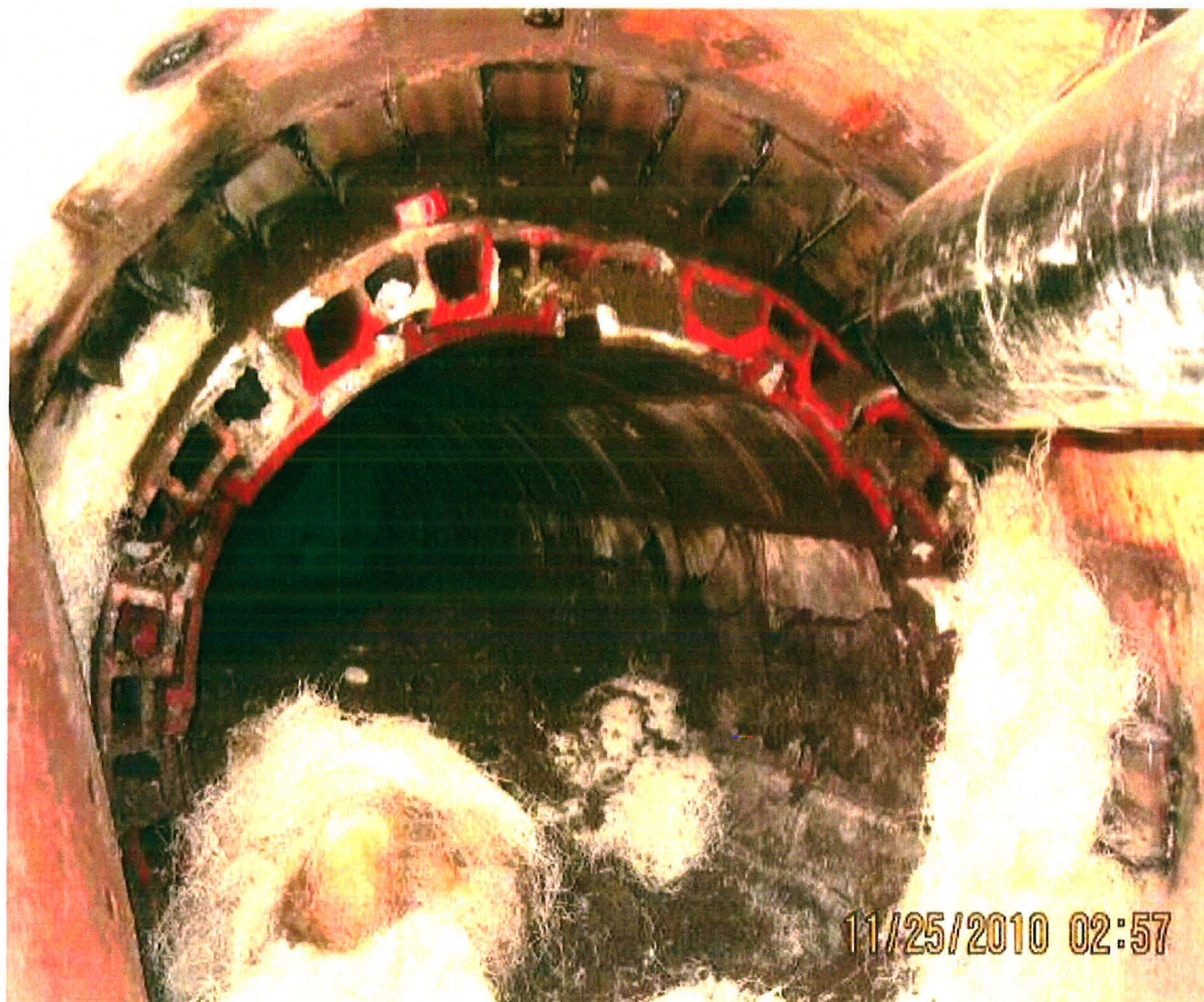
36-inch waterline at SE Foster Rd. Photo taken by Emery & Sons.
