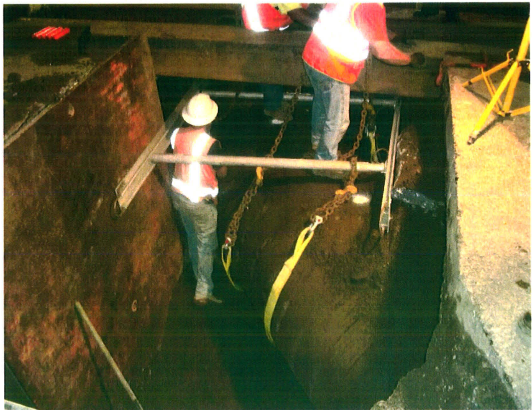
Installing straps on 60- inch water main support system.
