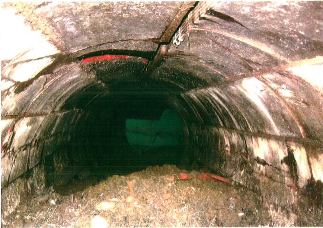
36-inch waterline on Foster
