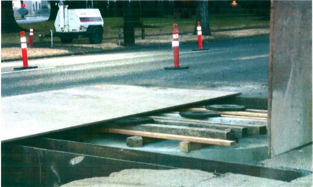
Placement of steel sheets after installation of Manhole 1.
