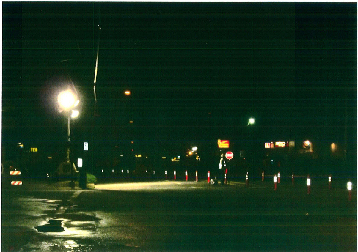
Traffic Control west bound Foster (Night time)
