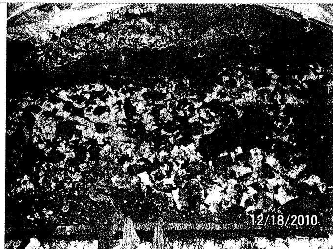
Figure 10: Grouted Zone at Beginning of Diggershield Excavation
