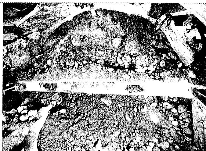
Figure 11: Ground Conditions at Front of Diggershield
