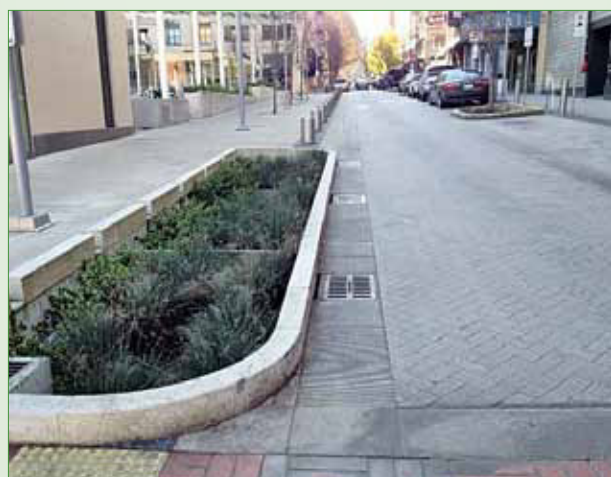
Flush tight sidewalk, SW 9th Avenue, Director Park
