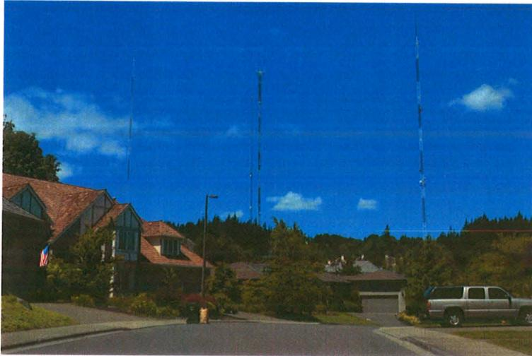
The tower farms along the Northwest Hills near Skyline Boulevard primarily broadcast digital television signals. These towers are generally 900+ feet in height and are classified as 'lattice style' supported by guy lines. Because of their height, they are required to have both the red and white aviation hazard paint scheme, as well as aviation hazard lighting.
