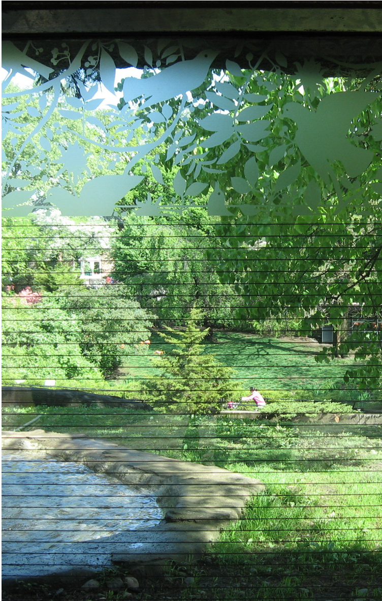
The window at the Philadelphia Zoo's Bear Country exhibit was the site of frequent bird collisions until this window film was applied. Collisions have been eliminated without obscuring views out. Photo: Philadelphia Zoo.
