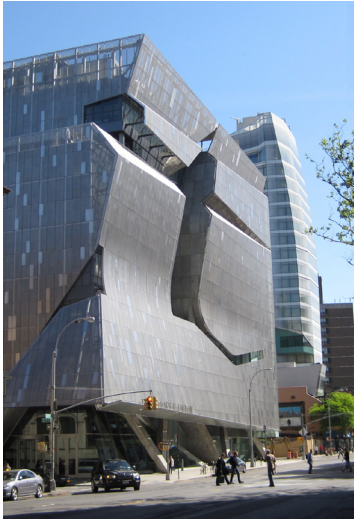
41 Cooper Square in New York City, by Morphosis Architects, features a skin of perforated steel panels fronting a glass/aluminum window wall. The panels reduce heat gain in summer and add insulation in winter while also making the building safer for birds. Photo: Christine Sheppard, ABC
