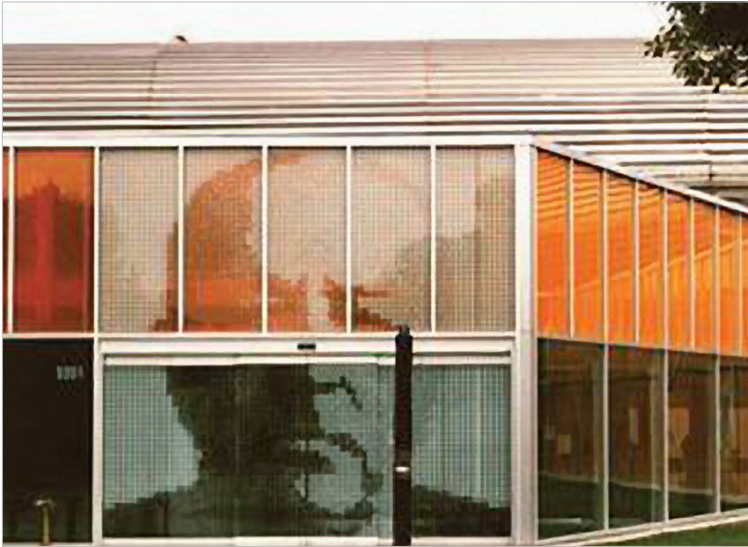
The IIT Student Center in Chicago uses faceted glass, Panelite panels and a dot matrix pattern (above) in its facade. These elements create visual noise which is perceptible to birds.
