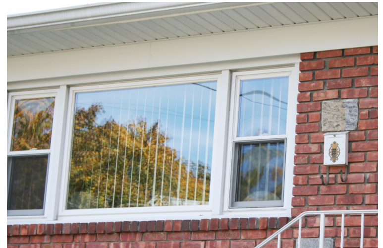
Reflections on home windows are a significant source of bird mortality. Partially opened vertical blinds may break up reflections enough to reduce the hazard to birds. Photo: Christine Sheppard, ABC
