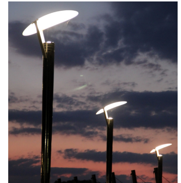
Cut-off shields can reduce lighting loss and permit use of lower wattage bulbs, resulting in lower costs. Shielded light fixtures are widely available in many different styles. Top photo: Susan Harder; bottom photo: Dariusz Zdziebkowski, ABC
