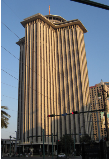
The World Trade Center of New Orleans, designed by Edward Durrell Stone, uses a simple bird-friendly strategy – almost all windows have exterior shutters. Photo: Christine Sheppard, ABC
