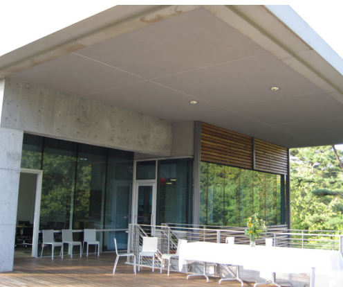
Overhangs block viewing of glass from some angles, but do not necessarily eliminate all reflections. Photo: Christine Sheppard, ABC
