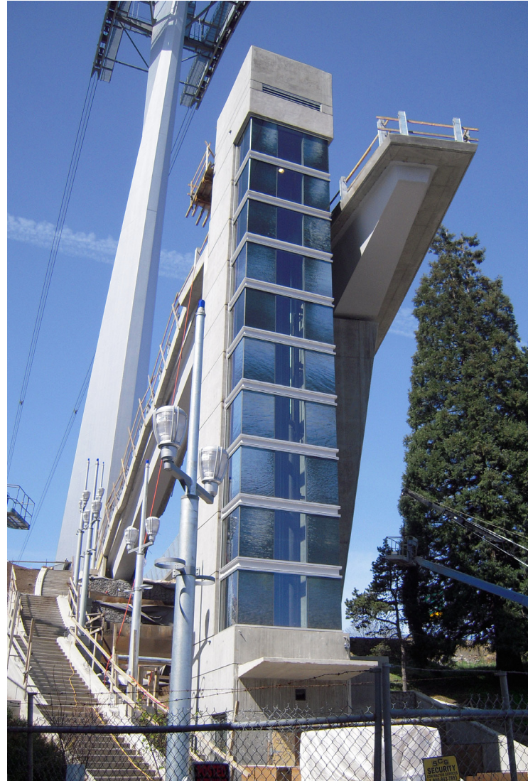
Fritted glass photo panels on the Gibbs Street Pedestrian Bridge elevator in South Waterfront are part of a public art project made possible by the Regional Arts & Culture Council and the Portland Bureau of Transportation through the City's Percent for Art Program. Artist Anna Valentina Murch made the photographs of water, which were printed onto the glass panels by Peters Studios, thus marking the windows for birds. Photo by Jeanne Galick.
