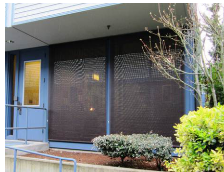
Six reflective windows on the Port of Vancouver administrative building are slated for a pilot installation of roll-up solar shades, which will serve the dual purpose of softening incoming light and reducing strike hazards. Top photo shows window with shades up and bottom shows the window with the shades down. Photo PoV.
