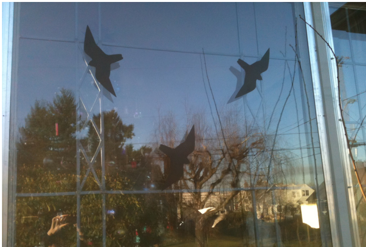
Silhouettes placed every 12 inches on the exterior of this residential window are spaced too far apart to reliably eliminate all strikes, but will likely reduce strike incidence.
