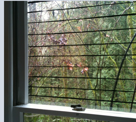
The view out of a window with horizontal tape spaced every 2 inches looks much like a view through miniblinds. Photos: Mary Coolidge
