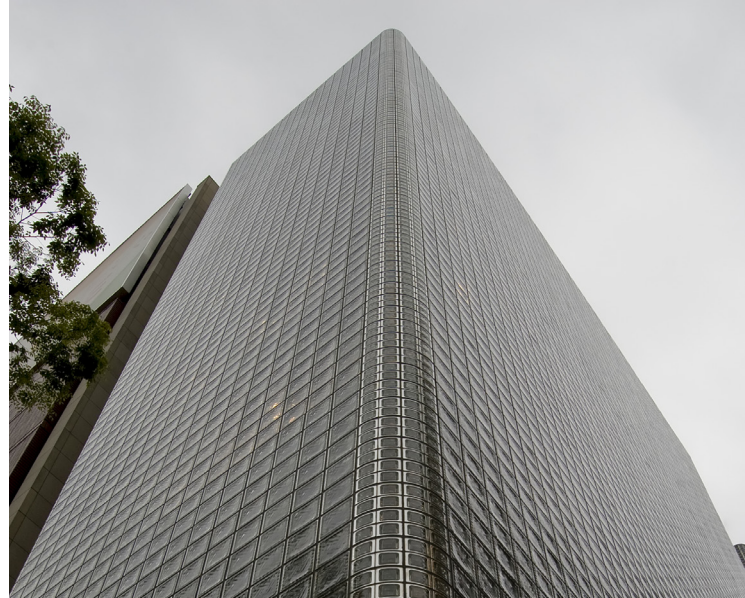
Renzo Piano's Hermes Building in Tokyo has a façade of glass block. Photo: Mariano Colantoni
