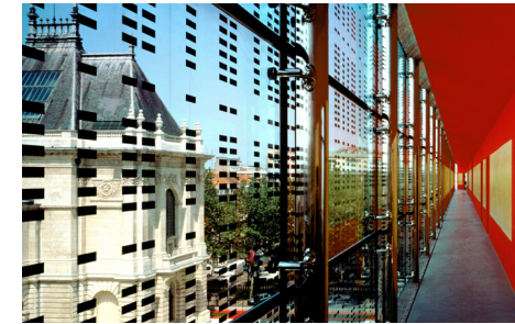
External frit, as seen here on the Lile Museum of Fine Arts, by Ibos and Vitart, is more effective at breaking up reflections than patterns on the inside of the glass. Photo: G. Fessy
