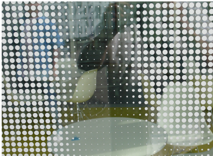
A detail of a pattern printed on glass at the Cottbus Media Centre in Germany. Photo: Evan Chakroff
