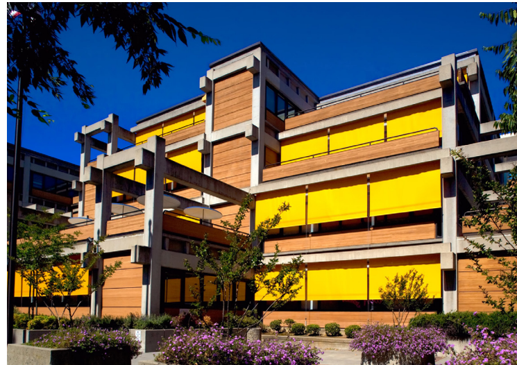
External shades, as shown here on the Batson Building in Sacramento, California, designed by Sym Van der Ryn, are a simple and flexible strategy for reducing bird collisions, as well as controlling heat and light. Photo: MechoShade
