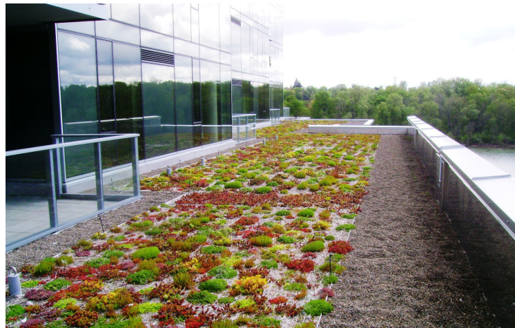
Unmarked glass adjacent to ecoroofs can be hazardous to birds that are attracted to available habitat. Photo by Tom Liptan
