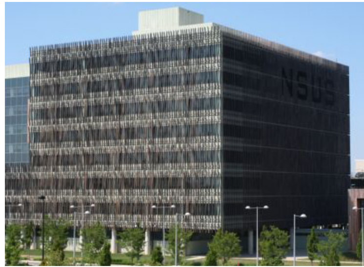
The U.S. Census Complex in Suitland, Maryland, designed by Skidmore, Owings, Merrill, features a brise soleil that shades the curtain wall. Wavy vertical fins of marine-grade, white oak reduce sun glare while eliminating glass reflections. Photo: Esther Langan
