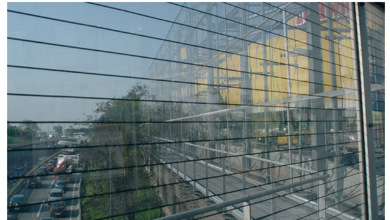
A pattern of narrow horizontal stripes has proven to be highly effective at deterring bird collisions, while covering only about 7% of the surface of the glass. Photo: Hans Schmid
