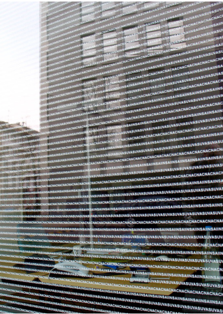
The glass facade of SUVA Haus in Basel, Switzerland, renovated by Herzog and de Meuron, is screen-printed on the outside with the name of the building owner. Photo: Miguel Marqués Ferrer
