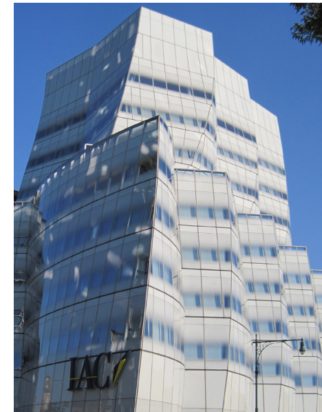
While some internal fritted glass patterns can be overcome by reflections, Frank Gehry's IAC Headquarters in Manhattan is so dense that the glass appears opaque. Photo: Christine Sheppard
