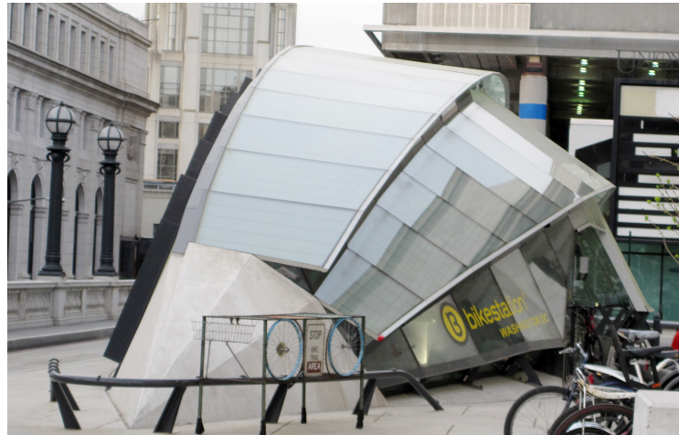
A dense internal frit pattern on the glass of the Bike and Roll building, near Union Station in Washington D.C., makes it look almost opaque. Photo: Christine Sheppard, ABC
