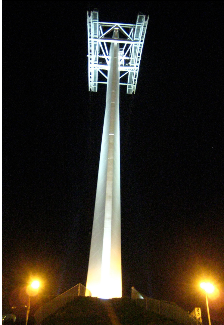
Unshielded, upward-directed floodlights at the base of the OHSU Tram Tower contribute directly to Portland's skyglow; existing fixtures which light the tram from above could instead be utilized as the primary lighting system. Photo: Mary Coolidge
