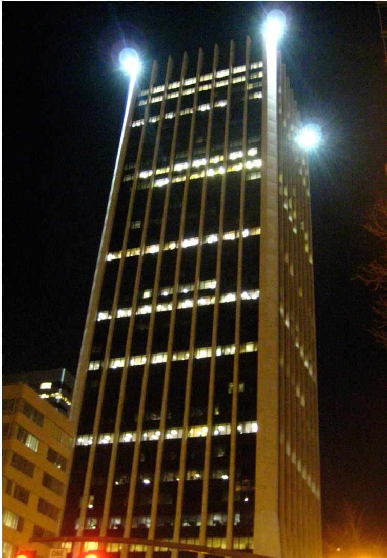
The height of the Wells Fargo Tower, coupled with its corner floodlights, make this building a potential collision hazard for migrants. Dimming or extinguishing exterior and rooftop lighting during migration season can help reduce collision hazards. Photo: Mary Coolidge
