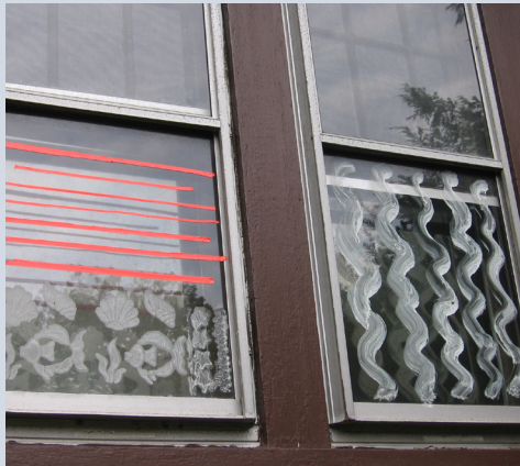
There are many quick, easy, and cost-effective ways to deter collisions on a short term basis. Here, tape stripes, stenciled, and free hand patterns in tempera paint on home windows. Photo: Christine Sheppard, ABC
