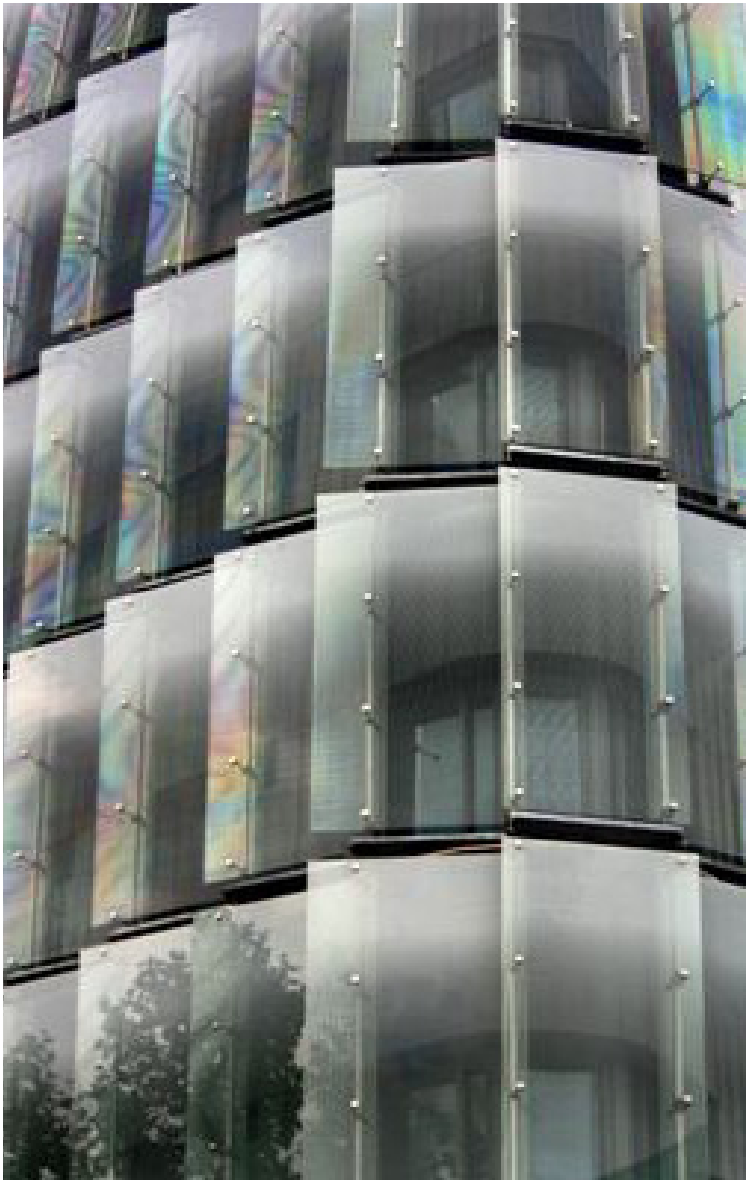
Galeo, part of a complex designed by Atelier Christian de Portzamparc in Issy les Moulineaux, France, has an external skin of printed glass scales which help to reduce reflections. Photo: Sipane
