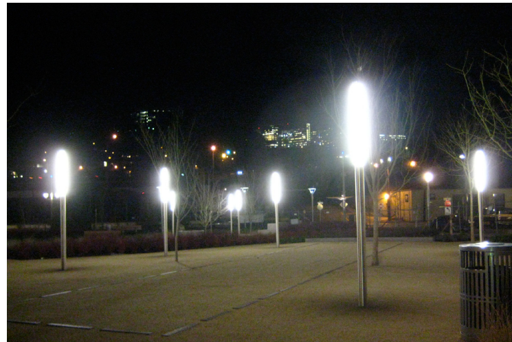
Unshielded lights in Elizabeth Caruthers Park in South Waterfront would benefit from full cutoff shielding to reduce contribution to ecological light pollution. Photo: Mary Coolidge
