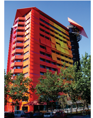
The Hotel Puerta America in Mexico City was designed by Jean Nouvel, and features external shades. This is a flexible strategy for sun control, as well as preventing collisions; shades can be lowered selectively when and where needed. Photo: Ramon Duran
