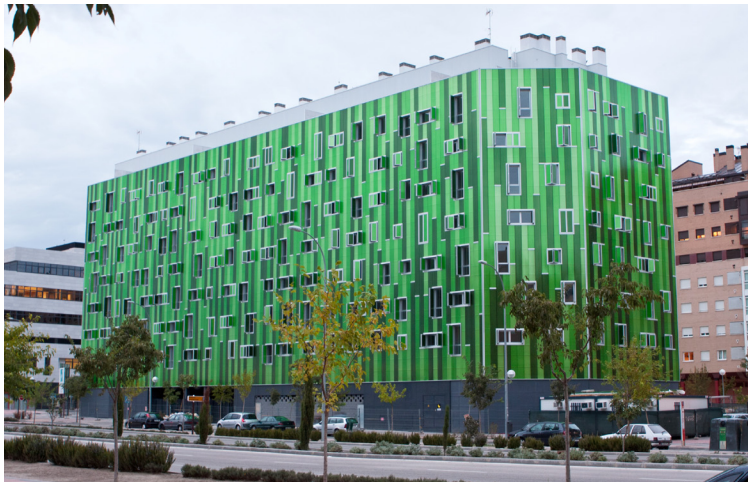
Madrid's Vallecas 51, designed by Somos Arquitectos, uses open-celled polycarbonate panels – a sustainable and recyclable skin that presents no threat to birds. Photo: Victor Tropchenko
