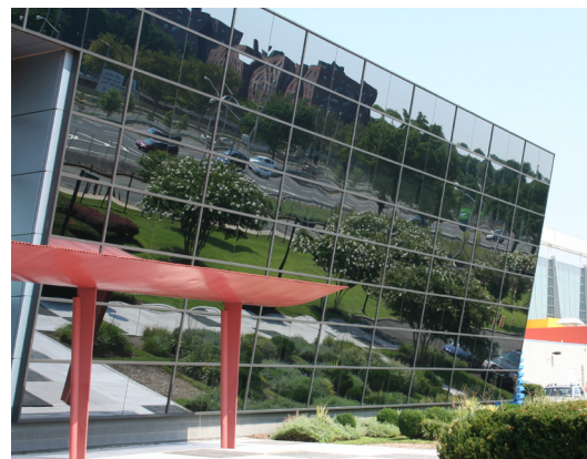
The angle on the New York Times printing plant facade is not sufficient to eliminate deceptive reflections of nearby vegetation. Photo: Christine Sheppard, ABC
