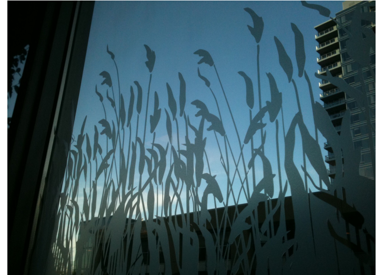
Privacy film on Mirabella windows preserves light entry and views out while marking the window for birds. Such film is more effective if applied to the exterior. Photo: Mary Coolidge
