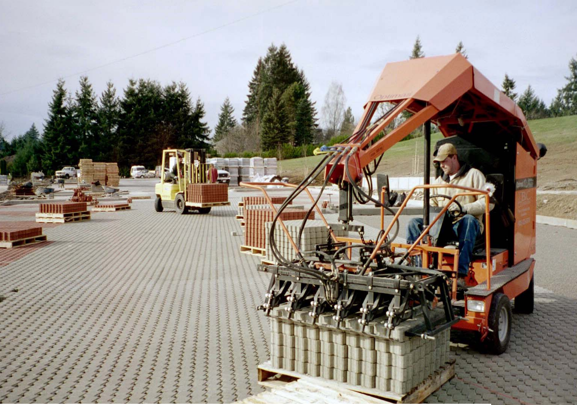
Installation of Eco-Loc Paver Parking Lot in Washington
