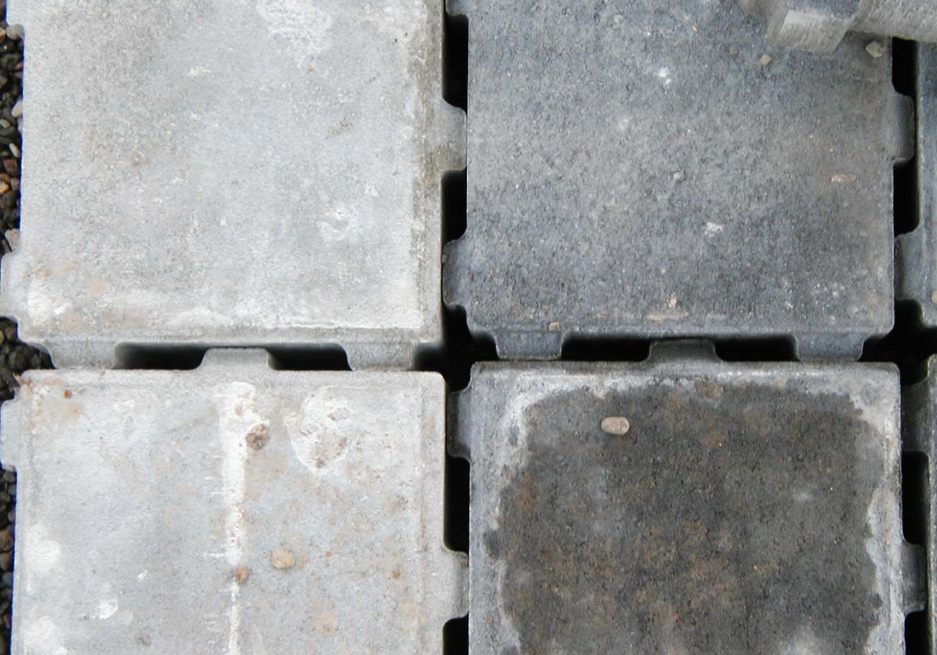
Pervious pavers at ONRC (5825 N. Greeley)
