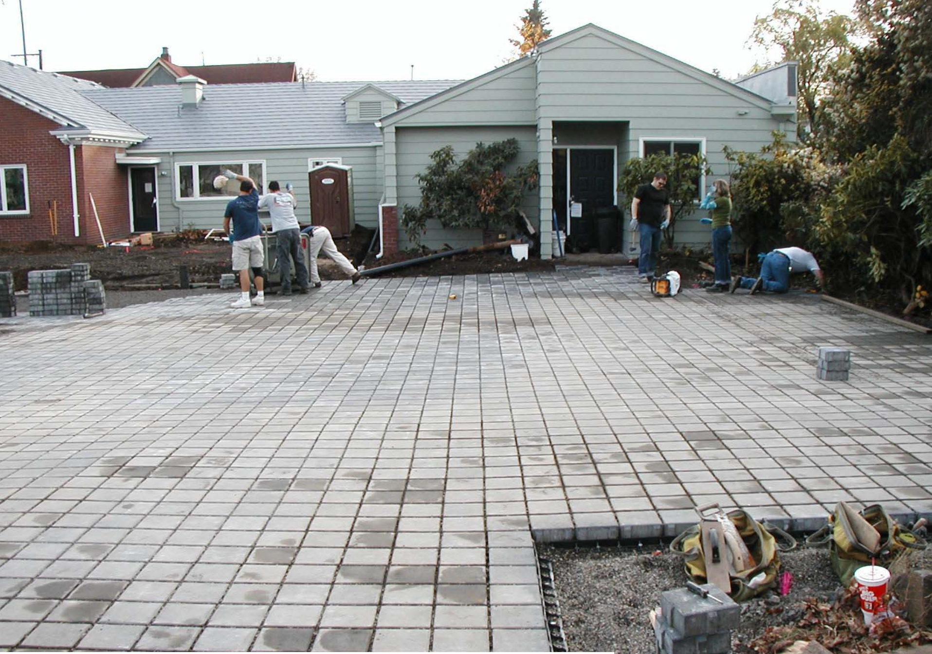
Pervious pavers at ONRC (5825 N. Greeley)
