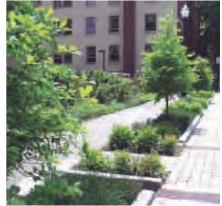
Vegetated filter box at SW 12th and Montgomery
