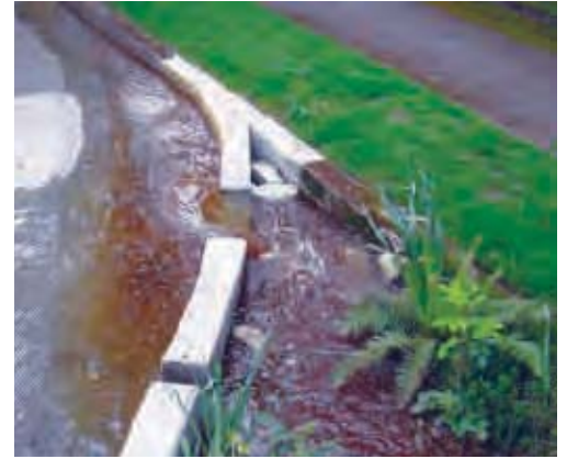
Curb extension at NE 35th Place and Siskiyou Street
