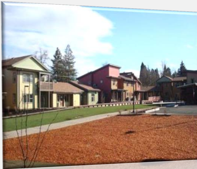
Bridge Meadows provides 27 units of intergenerational affordable housing.
