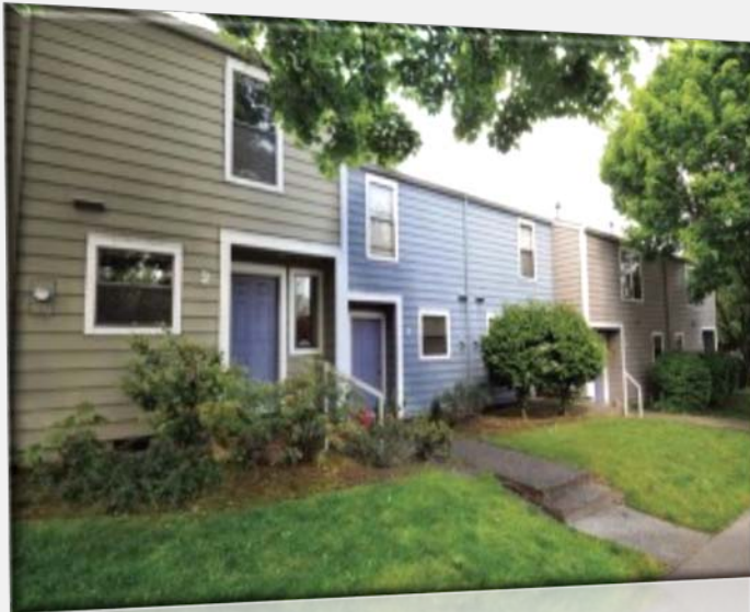
The Upshur House provides 30 units of affordable rental housing for families with less incomes less than 50% AMI. Address: 2650 NW Upshur St
