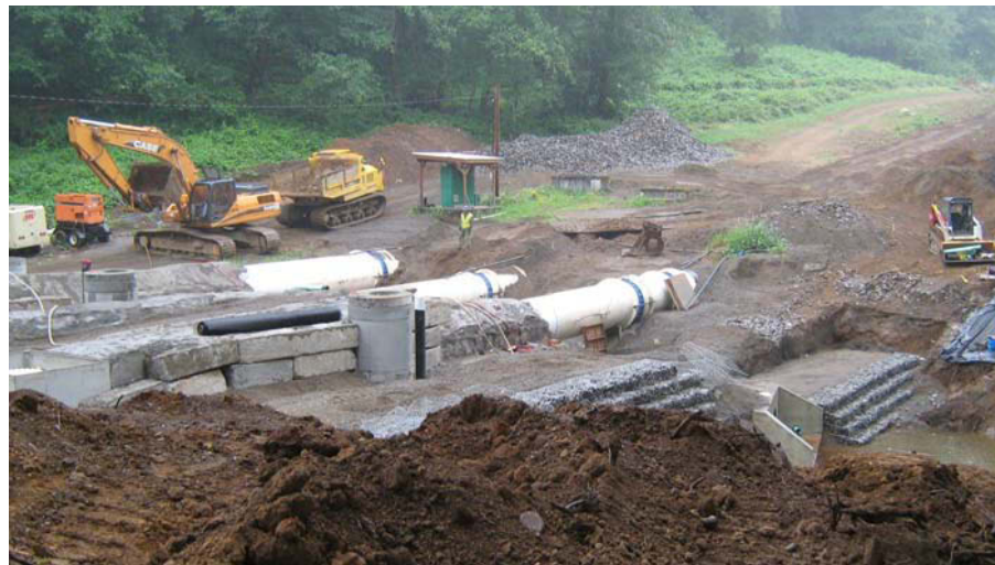
Seismic upgrades at Diack's pond
