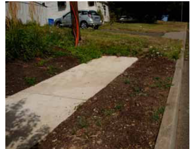
Street in Southwest. Sidewalk ends abruptly. Current regulations require new developments to include sidewalk improvements in the R.O.W. abutting the property.
