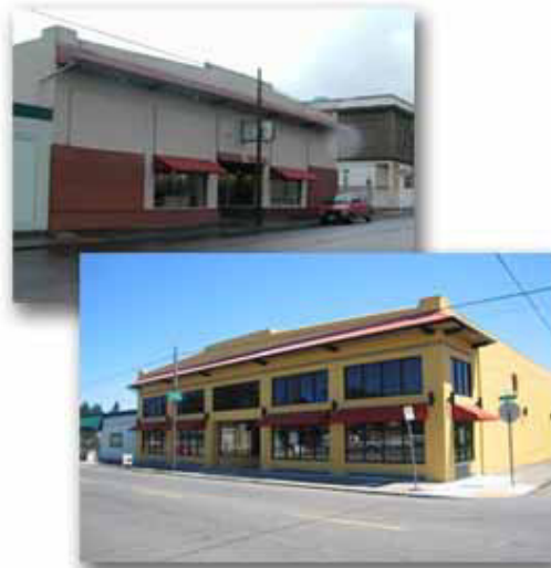
Historic facade at 5716 SE 92 nd Ave. in Lents, renovated through PDC's Storefront Improvement Program.
