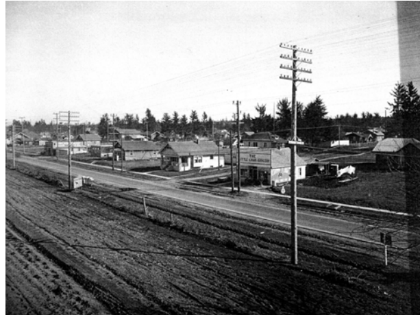
Lower density residential and commercial development across from agricultural land along NE Sandy, 1924. OHS image.
