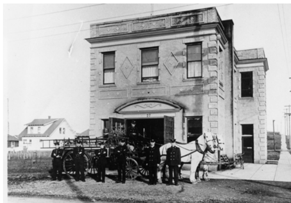
Fire house and Engine No. 272 on NE 82 nd Ave., 1913-1953.
