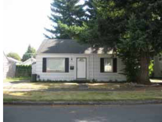
House constructed in 1944, SE 88 th and Alder.
