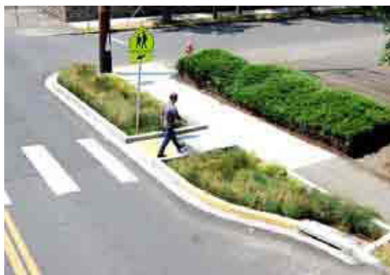
Stormwater curb extensions
