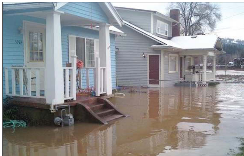
SE 104 th Avenue, Flood of 2009
