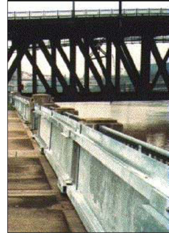
Flood protection barrier
