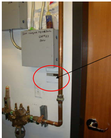
Figure 5-4b Furnace Room Temperature Sensor at Portland Parks Bureau Pittock Mansion Tea House
