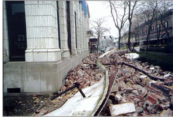
Unreinforced masonry building debris from M 6.8 Nisqually Earthquake, 2001
