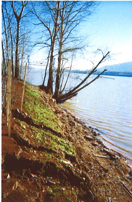
BES Lab: Bioengineering Failure – Compost Soil and plants floated away (1995-1996)
