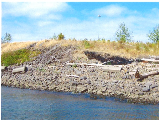
Failed Bioengineering on Willamette – Erosion exposed GEOTEXTILE Fabric 2009
