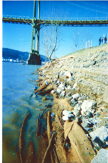
BES Lab: Bioengineering Failure – Compost Soil and plants floated away (1995-1996)
