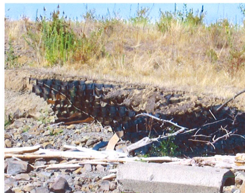
Failed Bioengineering on Willamette – Erosion exposed GEOTEXTILE Fabric 2009
