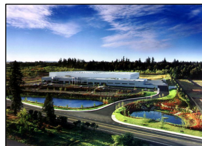
Ford's Rouge Center truck plant in Dearborn Michigan includes a 10-acre ecoroof.
