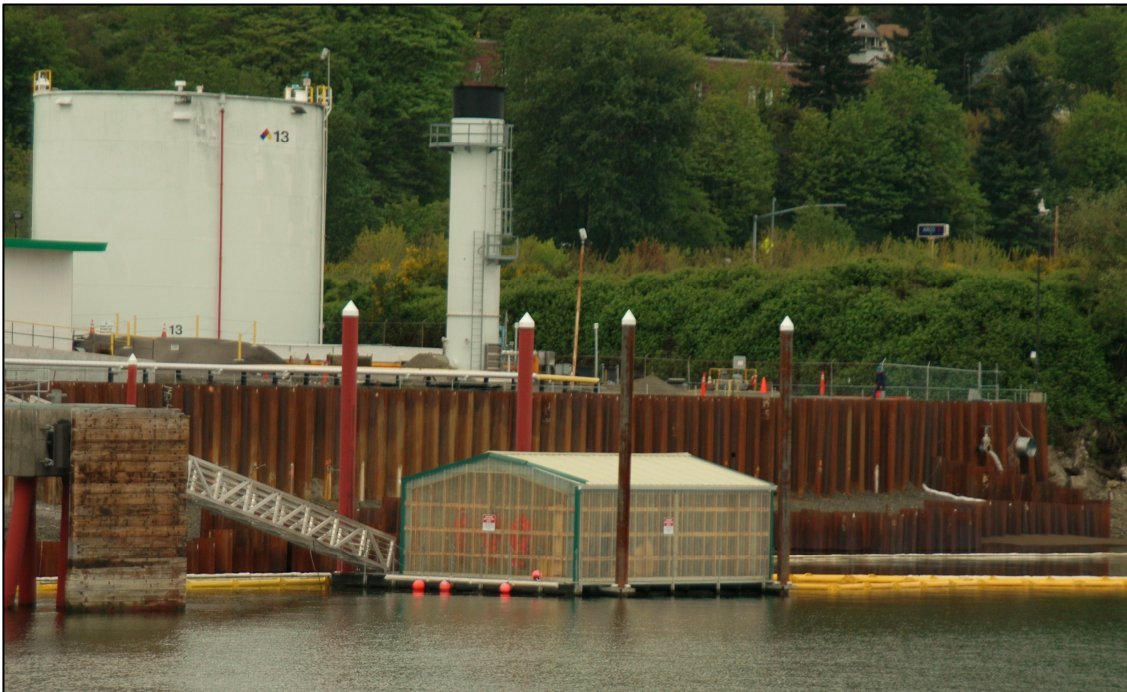
The River Plan aims to reduce permitting time for projects like the new sheet pile wall at the BP facility.
