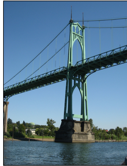
The majestic St. Johns Bridge soars above the North Reach of the Willamette River.
