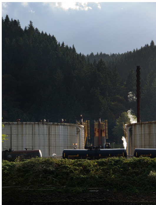
The petroleum cluster is a critical element of the harbor's industrial economy.
