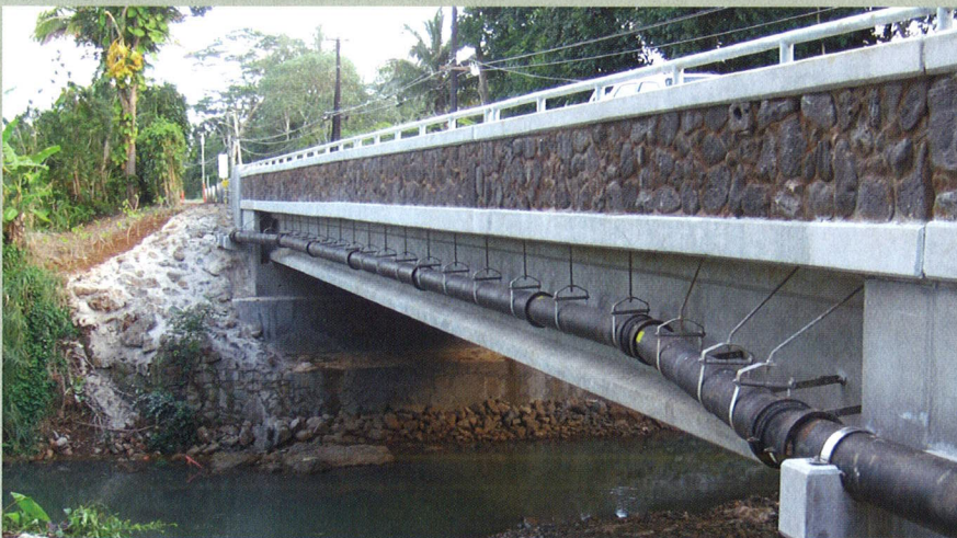
A "soft opening" ceremony opened the Kilauea Stream Bridge to traffic December 4, 2008, nearly three months ahead of schedule. A traditional Hawaiian blessing ceremony was held with state-level dignitaries on hand December 19 to officially open the bridge.
