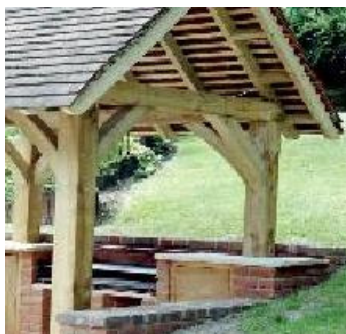
These amendments code establish setbacks, height and building coverage for structures in common tracts.
